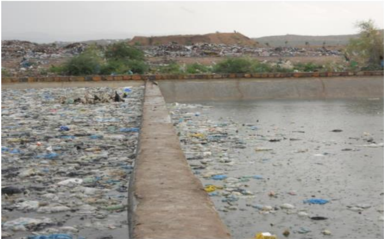
Figure 18 Dire Dawa landfill site, showing cell having solid waste mixed with liquid
