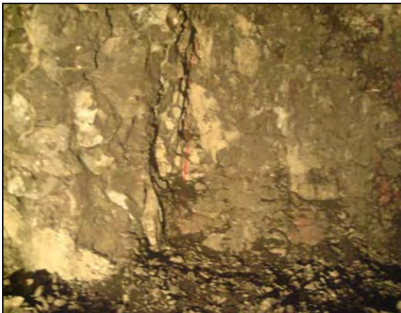
Fracture line on weathered breccia rock unit
