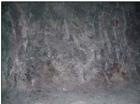
Massive breccia unit (no pronounced joints)
