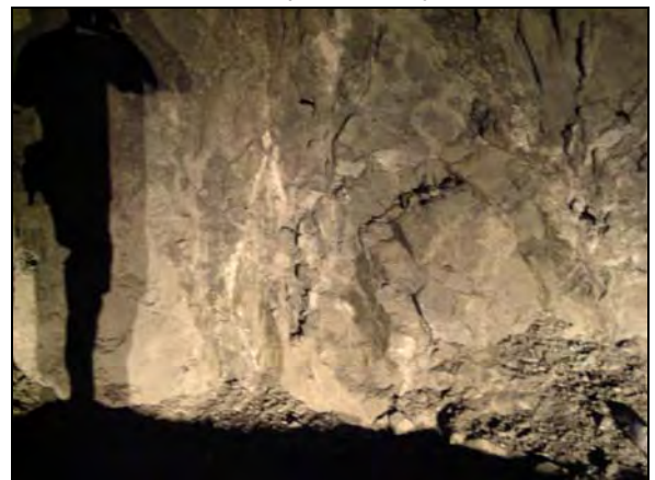
Weathered and fractured breccia unit on draft tubes
