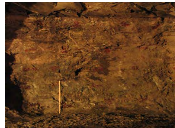
Slightly weathered breccia with rough surface (no considerable joint sets)
