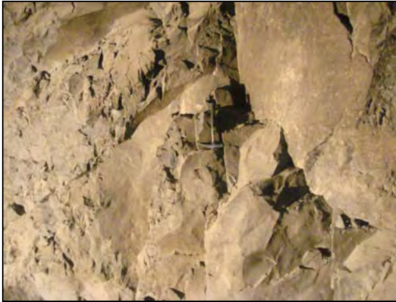
Two joint sets with smooth joint surface in Aphanitic basalt
