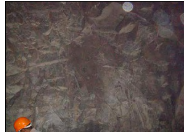
Fractured Aphanitic basalt in a bus duct gallery
