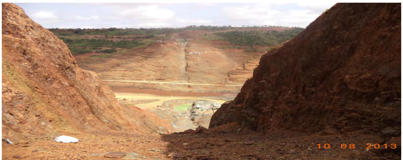
Picture – 3.1 Trench along the dam axis of study area
