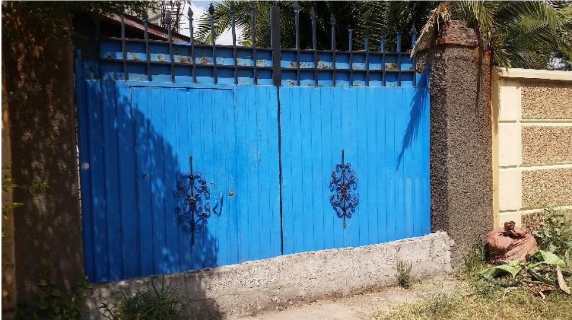
Figure 9: Image showing a retaining wall-like structure with a hollow block to defend flooding.
