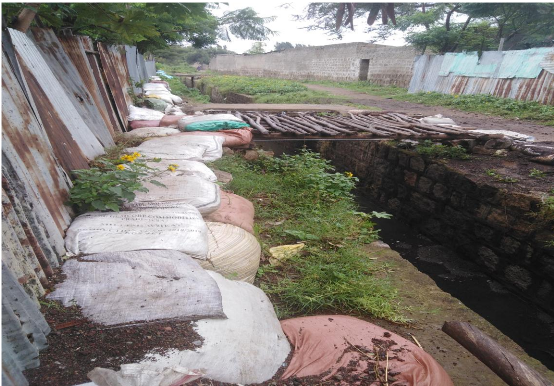
Figure 8: Shows sandbags as a blockage of flooding water.
