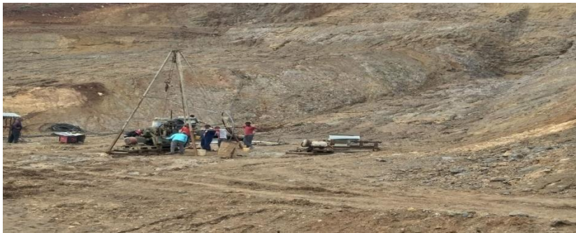
Figure 5.11 Grouting test in Weak formation at left abutment
