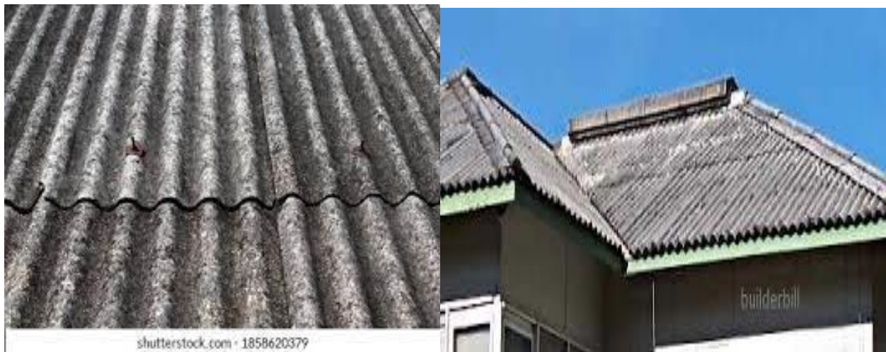
Figure 2. 1 Asbestos cement corrugated roof
