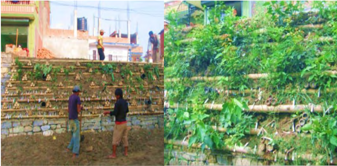
Figure 25: The vegetated bamboo crib wall just after construction (November 2006) and after one year of construction (Kusunti, Lalitpur, November, 2007)
