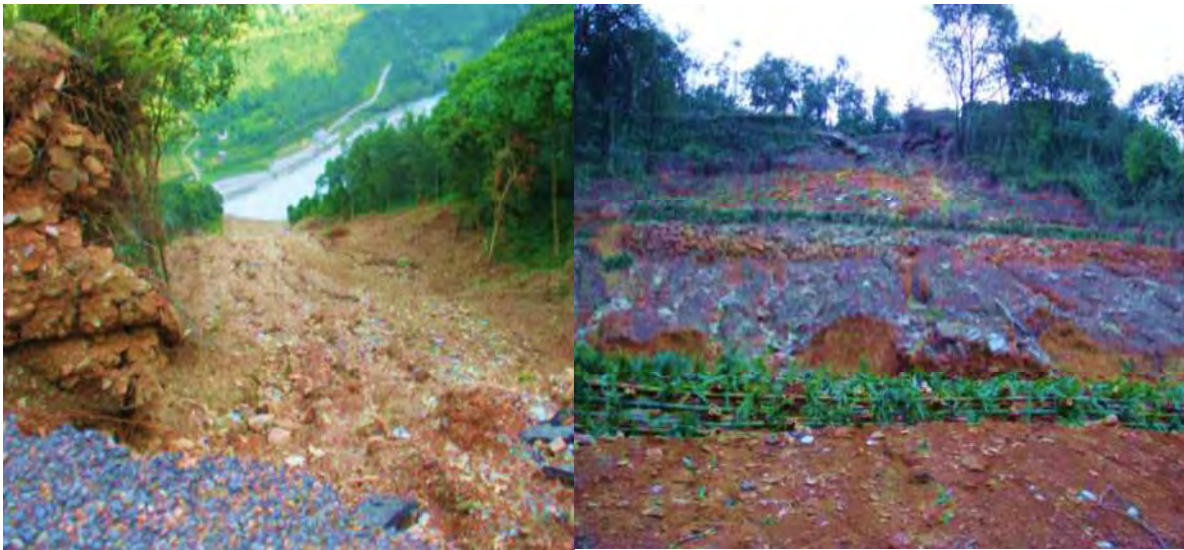
Figure 28: Before and after construction photographs, Sarangkot landslide, Pokhara (January, 2008)
