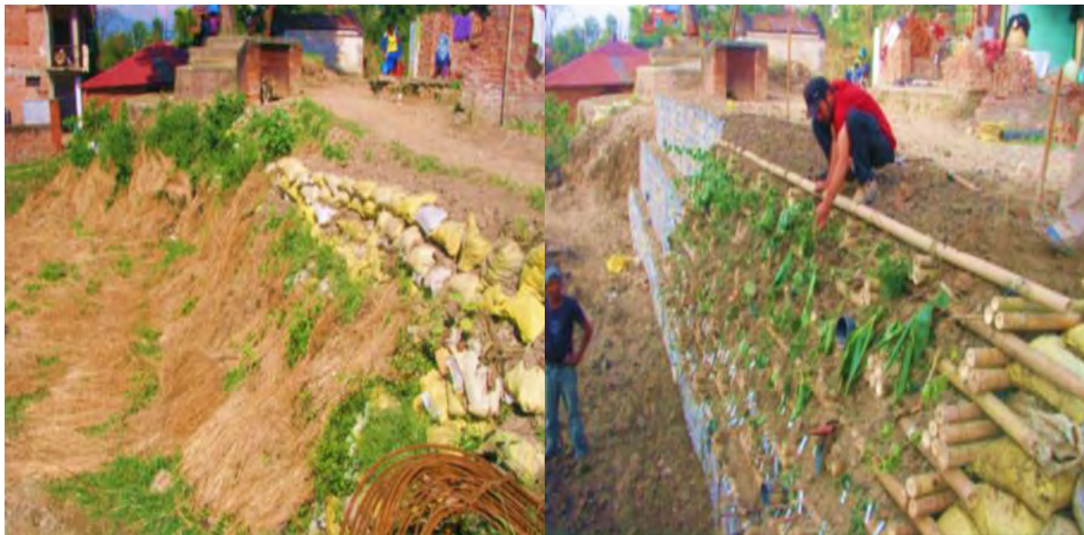
Figure 24: Before and after construction photographs, Kusunti, Lalitpur [28]
