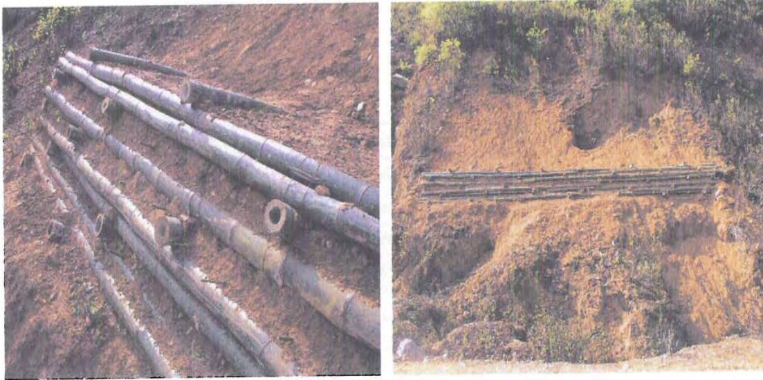
Figure 29: Vegetated bamboo crib wall construction in Thankot [30]
