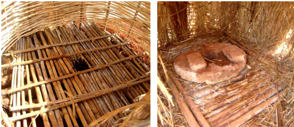
Figure 7: Common bamboo pit latrine structures used in Assosa rural settlements
