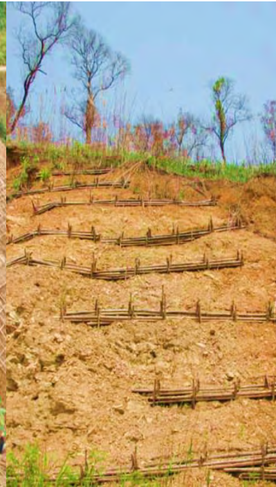
Figure 21: The bioengineering works remained stable even during fierce monsoon rains in 2007
