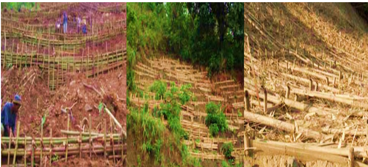
Figure 18: Bamboo terracing, bamboo crib walls, and bamboo knitting were developed to suit the requirements of each slope [24].
