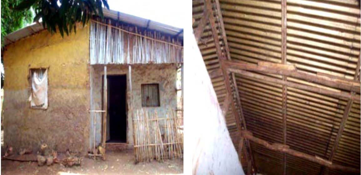
Figure 12: Front elevation and roof of the traditional-modern house in Assosa
