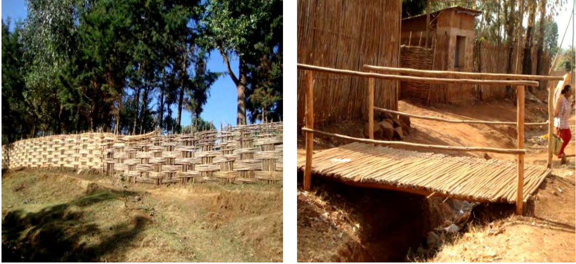
Figure 10: Use of bamboo as a fencing and bridge material
