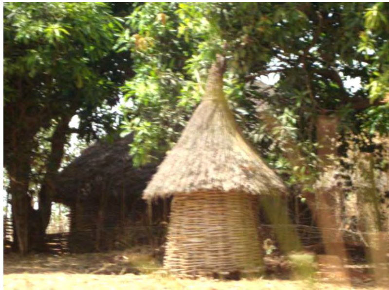
Figure 11: Bamboo as a building and construction material for grain storage granary in Assosa
