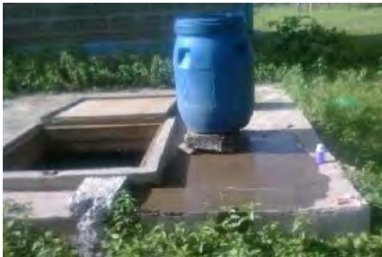
Plate 3.3 Constant-head drip chlorinator A 500m 3 Water tank
