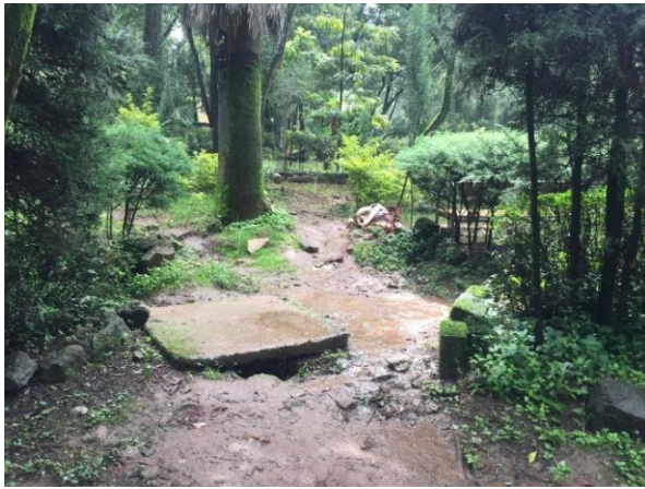
Figure 47: Open manhole on the travel path at Yeka Park (Left) and open drainage on the travel path at Beheretsige Park (Right). (Source - Author)
