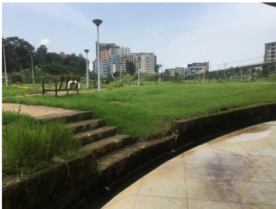
Figure 45: Stair with no landing and leading to an open drainage at ECA Park (Left) and open manhole on the travel path at Beheretsige Park (Right). (Source - Author)
