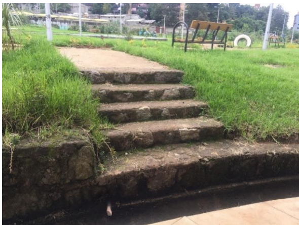
Figure 24: Stair falls into an open ditch with no proper landing at ECA Park (left) and Stair with no regular riser and trade at Addis Ketema Park. (Source - Author)
