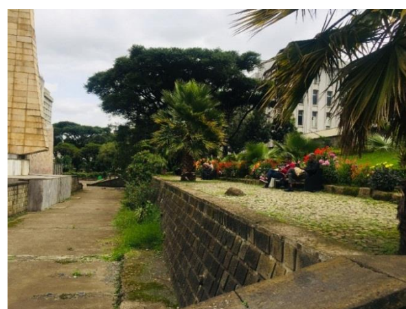
Figure 49: Elevated Path ways from adjacent landscape with no Protective rail or curb at ECA Park (Left) and ramp with no landing and protective handrail at Ethio Cuba Park (Right). (Source - Author)
