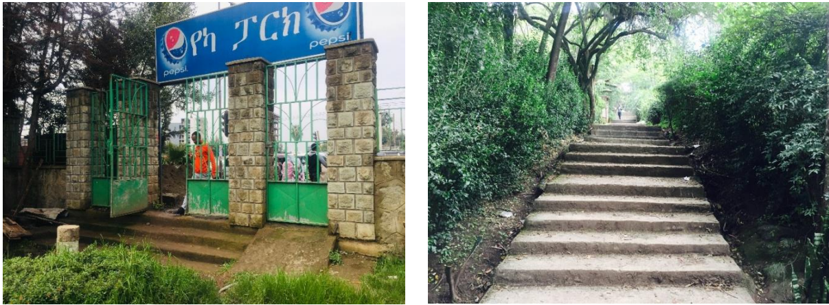
Figure 26: Stair with alternative ramp at Yeka Park (left) and, Stair with no Provision of ramp at Beheretsige Park (right). (Source - Author)
