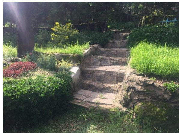
Figure 24: Stair falls into an open ditch with no proper landing at ECA Park (left) and Stair with no regular riser and trade at Addis Ketema Park. (Source - Author)
