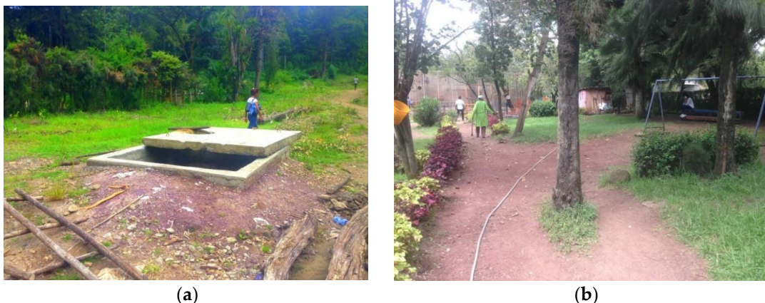
Figure 3. (a) Open manhole on the travel path at Beheretsige Park; (b) Tree planted on path of travel at Beheretsige Park. (Source - Author)
