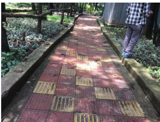
Figure 15: Misplaced tactile marking in Pathways at Yeka Park (left) and Damaged Pathways at Beheretsige Park (riahht). (Source - Author)
