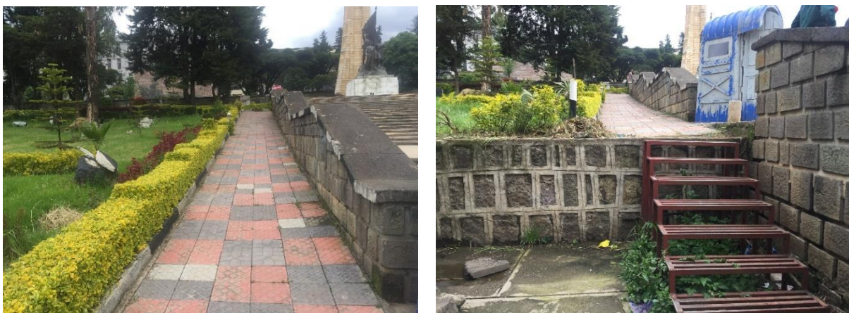
Figure 20: Terrazzo paved ramps with protective hand rail at the side but dropping to a stair with no safety consideration at Ethio - Cuba Park. (Source - Author)
