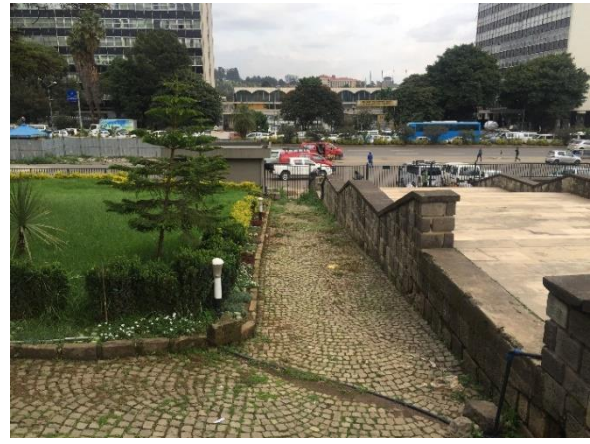
Figure 21: Cobble stone paved Ramps with no protective hand rail, no landing and damaged at Ethio - Cuba Park. (Source - Author)
