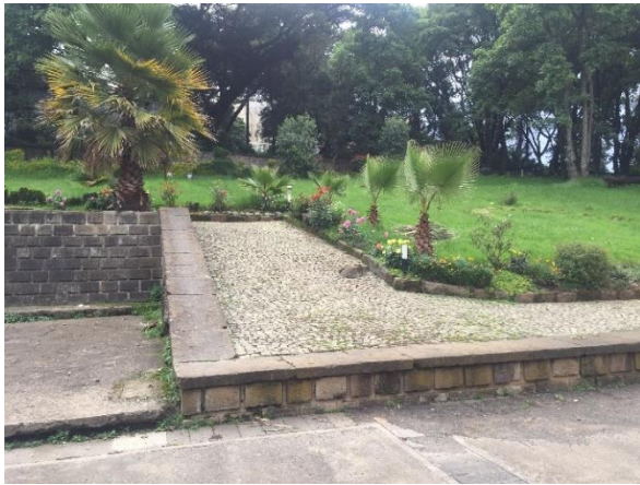
Figure 21: Cobble stone paved Ramps with no protective hand rail, no landing and damaged at Ethio - Cuba Park. (Source - Author)
