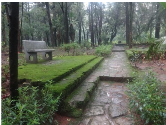
Figure 25: Stair grown alga at Peacock Park (left) and Stair with a width above 3000mm but no intermediate handrail at Ethio – Cuba Park. (Source - Author)
