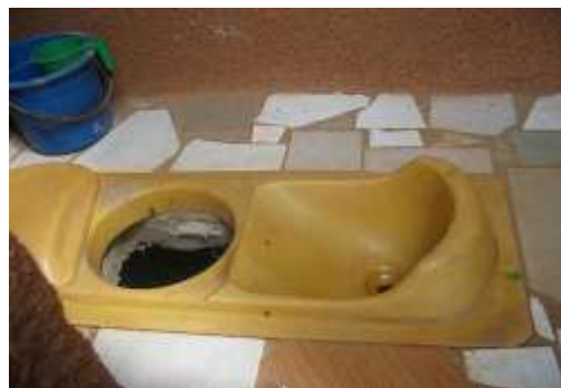
Figure 2 Urine diversion dry toilet (UDDT) internal design (left) a squatting type of UDDT Source: (Rieck et al. , 2012).
