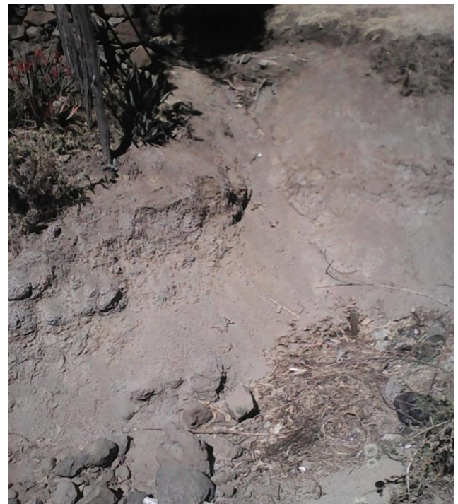
Plate 3. 7 Mikawa river bank failure
