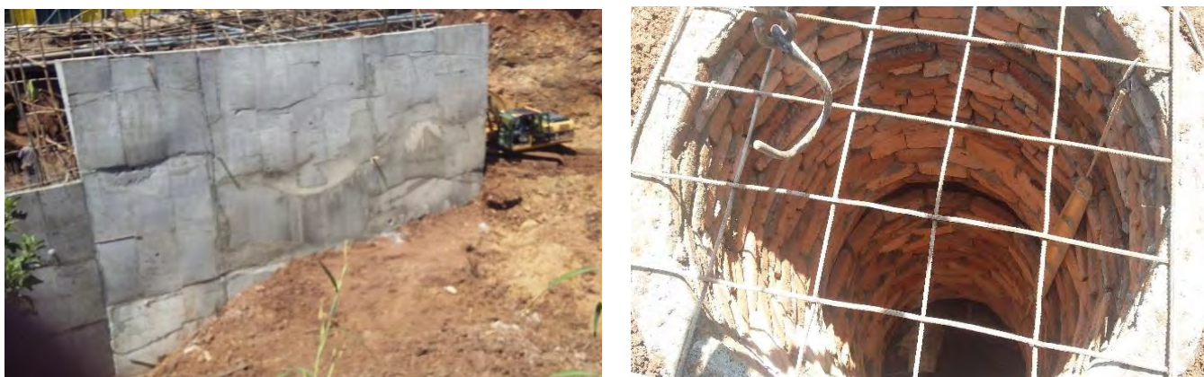
Figure 4.12: Construction of retaining wall
