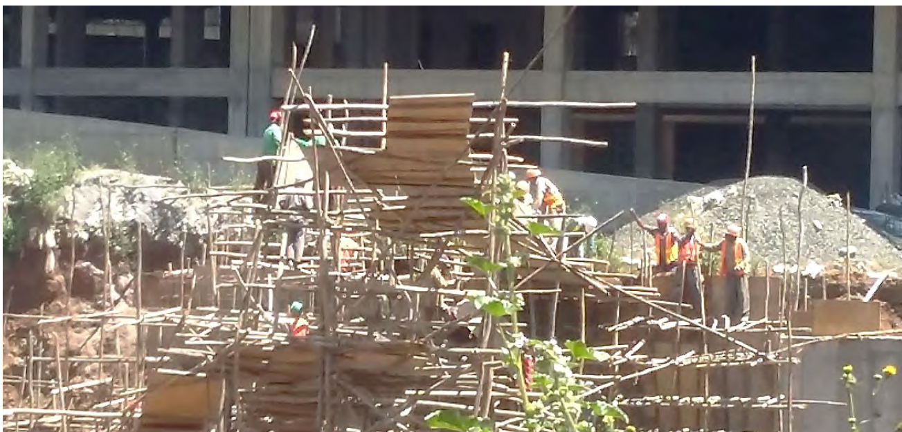
Figure 4.22: Construction of protection wall to avoid future sliding & to protect the neighbor structure
