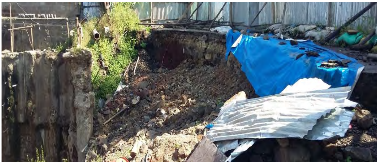
Figure 4.18: Effect on neighboring structure; collapse of feeder road
