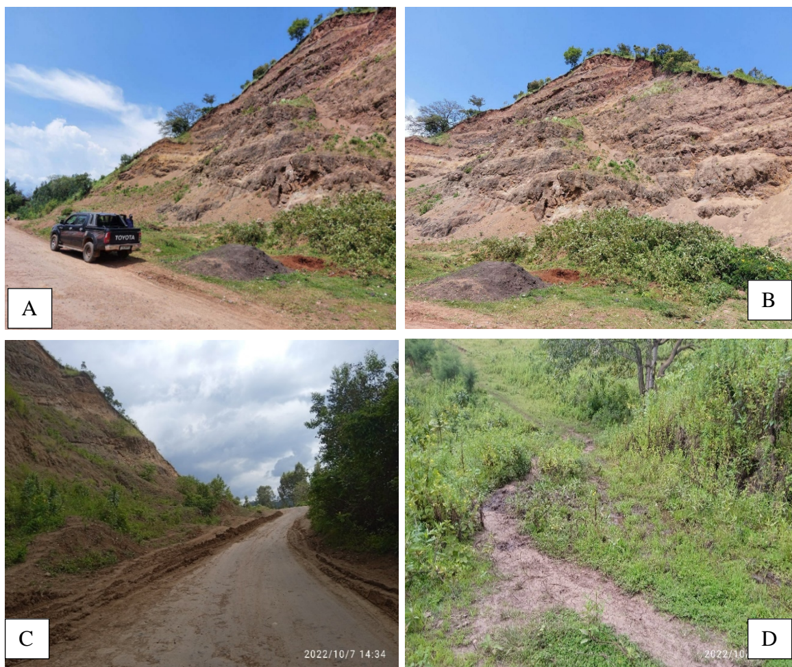
Plate 4-11: Landslide at site JC/S/11: A-C steep back slope material of highly weathered and fractured basalt. D)Swampy area at right hand side of the downslope.
