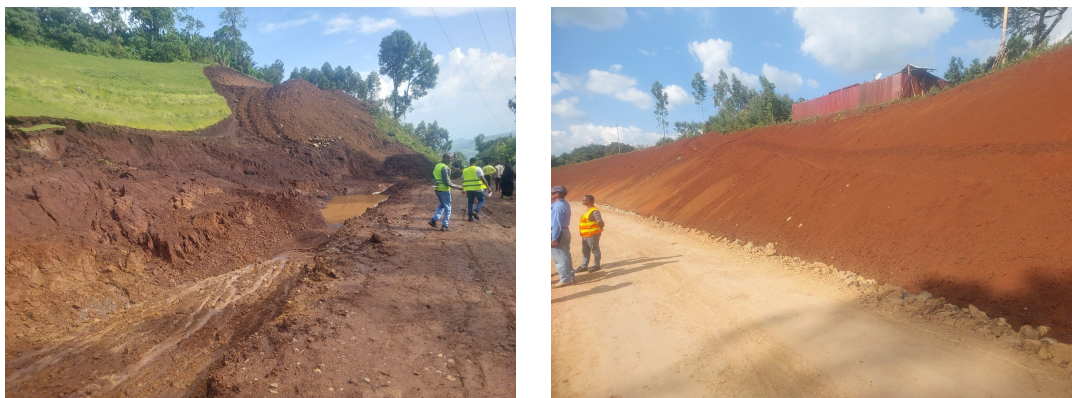
Figure 3-9: Residual soil along the road mostly covering the flat and rolling part of the corridor.
