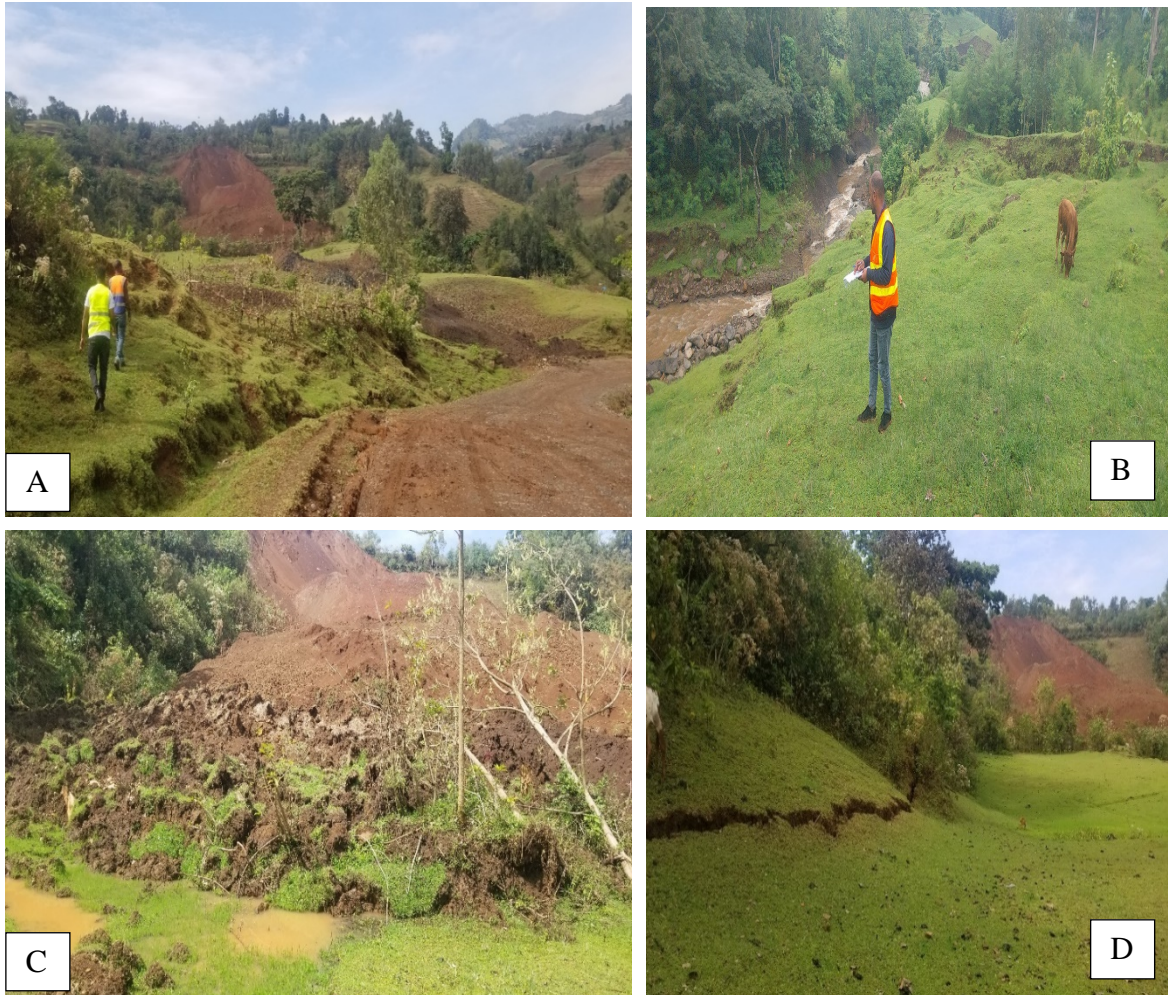
Plate 4-1: Landslide at site JC/S/01 A) Spoil mass triggering the landslide B) Slide mass toward the stream at the toe C)Wet area due to multiple springs D)Long tension cracks developed by moving mass.
