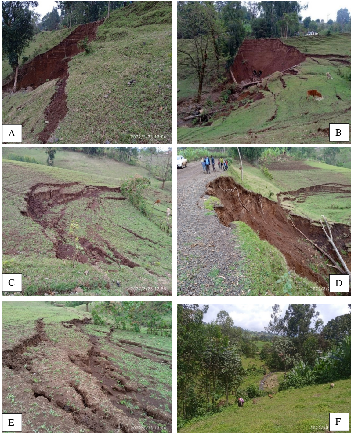
Plate 4-9: Landslide at site JC/S/09: A)Landslide of road side slope B)Typical rotational landslide of the slope C)Cracks developed at the side slope of the road D)Landslide propagating towards the road corridor E)Moving slope mass F)Upstream side of the landslide section.
