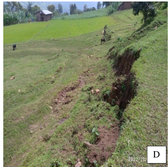
Plate 4-6: Landslide at site JC/S/06: A)The main scarp on the back slope B)Springs on the back slope C)Landslide area covered by trees D)Destabilized side slope on the left hand side of the road.
