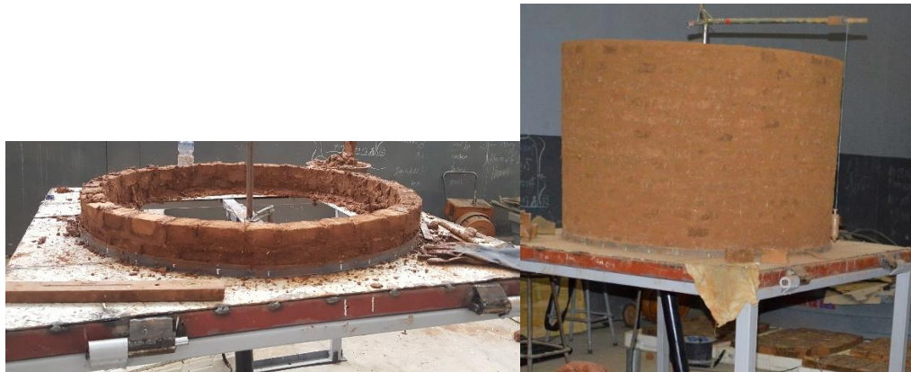
Figure 4-19 construction of the model
