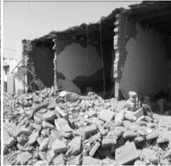
Figure 2-14. Out-of-plane failure.
