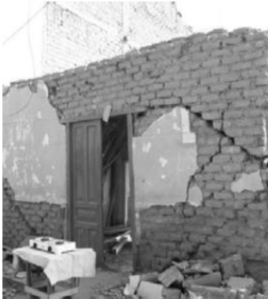
Figure 2-13 In-plane failure.
