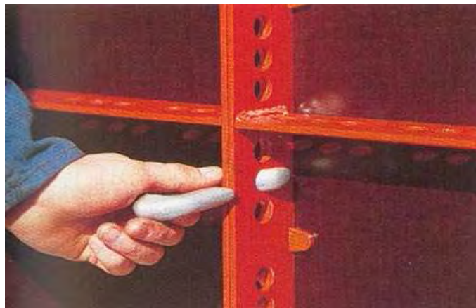
Figure 3.10 HANDSET wall formwork and its clip
