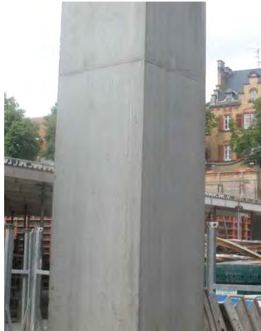
Figure 4.10; Concrete column formwork casted using PERI formwork, Darmstadt
