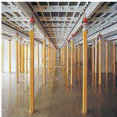
Figure 3.17 large prop spacing (left) and erection and lowering of drop head (right)
