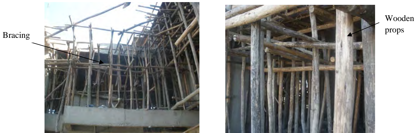
Figure 2.6 Slab formwork construction systems in Addis Ababa.
