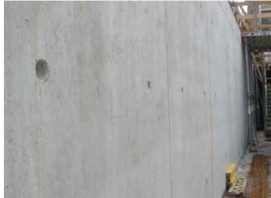
Figure 4.9 Concrete surface casted using TRIO panel, Darmstadt
