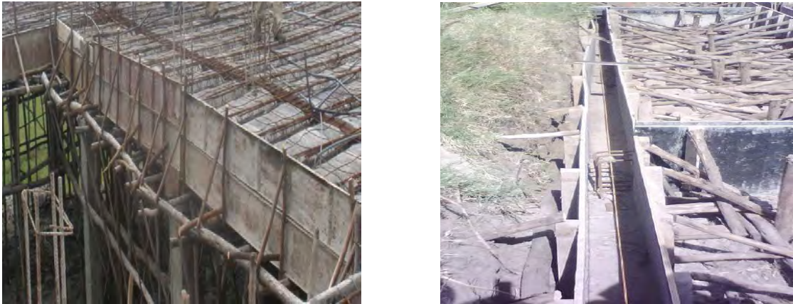
Figure 2.7 Beam Formwork Construction Systems in Addis Ababa.
