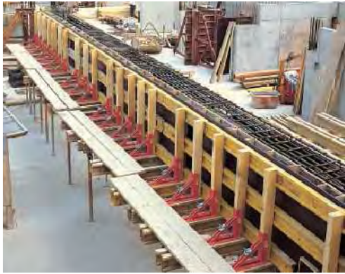
Figure 3.22 UZ beam formwork with its bracket and perforated rail
