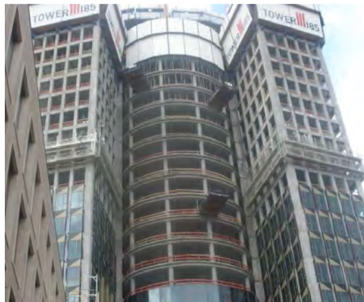
Figure 4.11 Self Climbing Systems at Tower 185, Frankfurt
