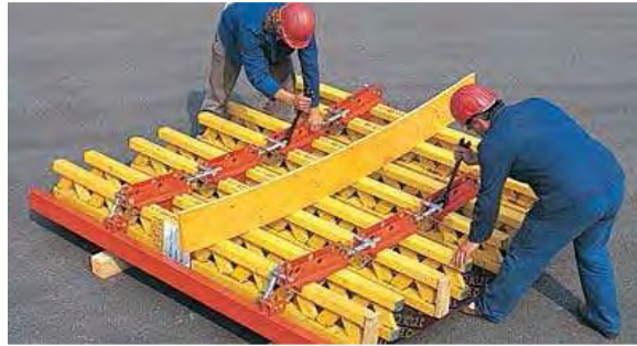
Figure 3.9 Adjustment of RUNDIFLEX
