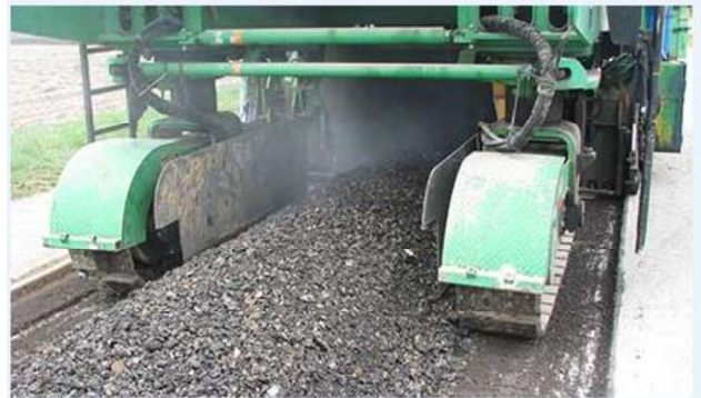
Figure 2-4: Cold in Place Recycling (CIR)
