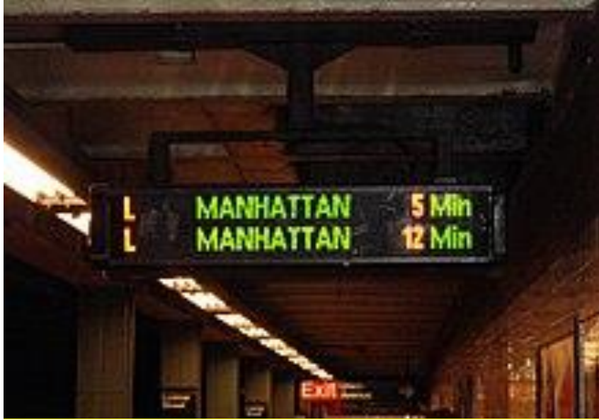
Figure 9 Typical Station Passenger Information System (New-York rail)
