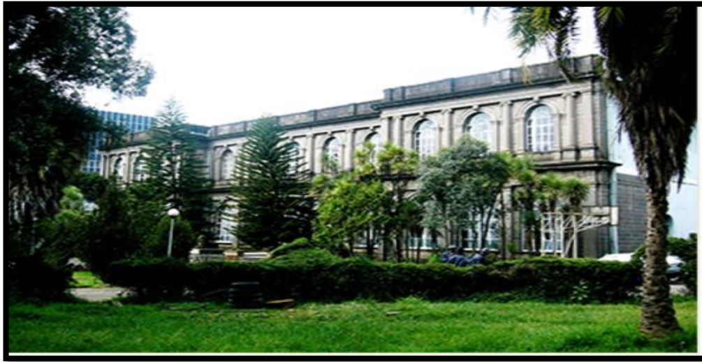
Kegnazmach Mekonen Endalkachewu Residence (Arada sub city)
