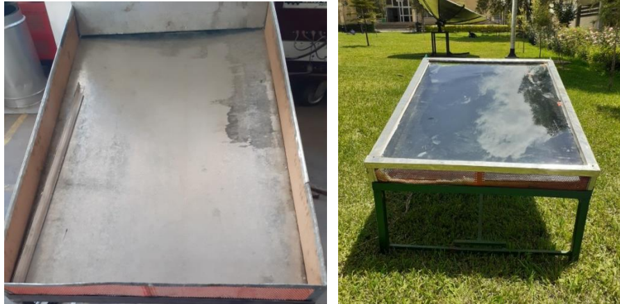
Figure 4.7- Assembly of solar collector for the tea dryer
