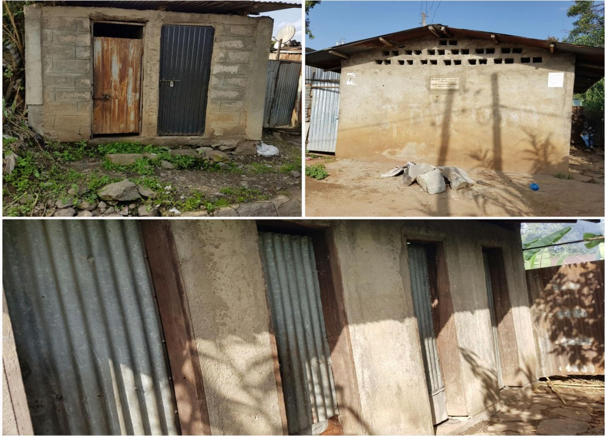
Photo: Sharing toilets in kebele 19
