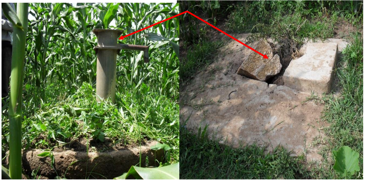
Plate 2. Abandoned and dismantled dry hand dug wells around the Haromaya dry lake well field.
