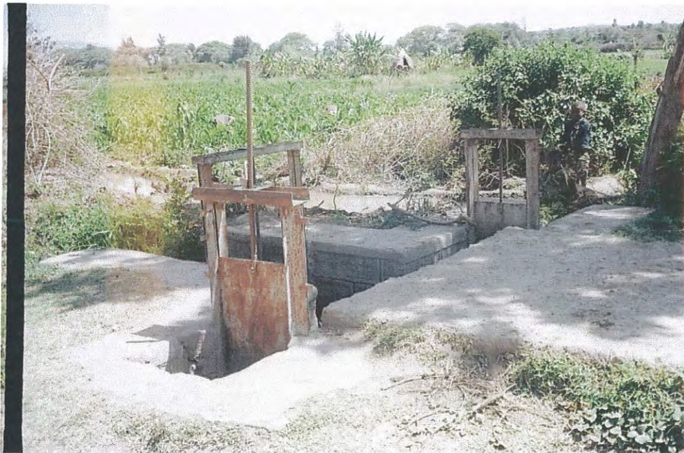
Figure 6: Main canal and Division boxes
