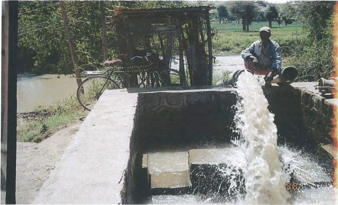
Figure 5: Delivery pool, only one of the pumps is operating
