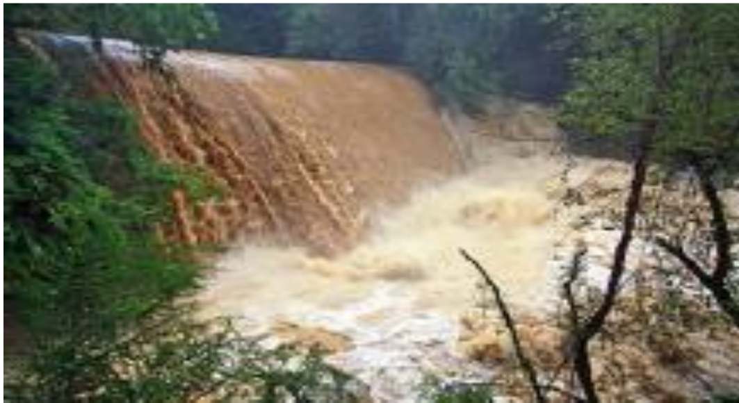
FIGURE 2.1: WATER OVERTOPPING THE MORGAN FALLS DAM
