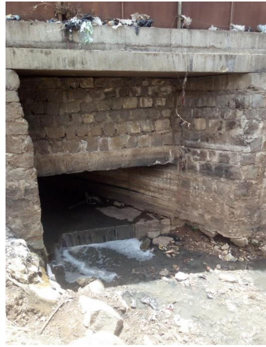
Figure 4.4: Exit of the Culvert
