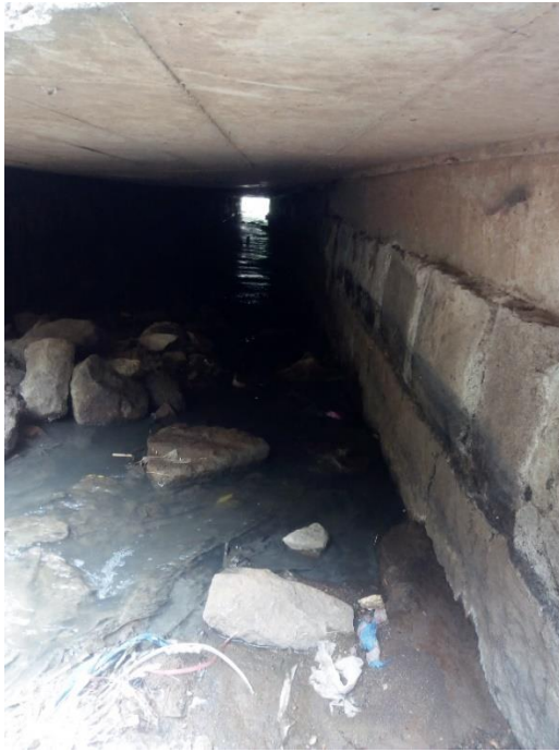
Figure 4.3: Entrance of the culvert
