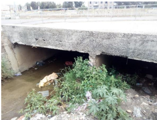
Figure 4.19: The two barrels of culvert on site
