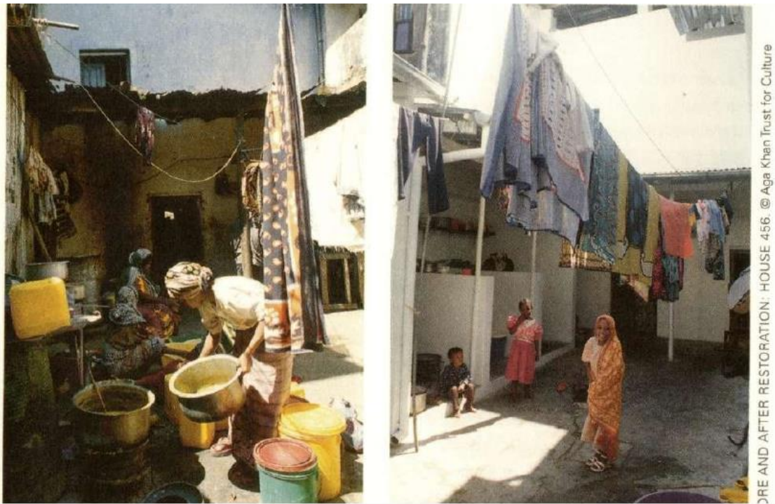
Figure 3-24 Upgrading of Communal Washing place, from Battle, Melin, and Forsman 2007
