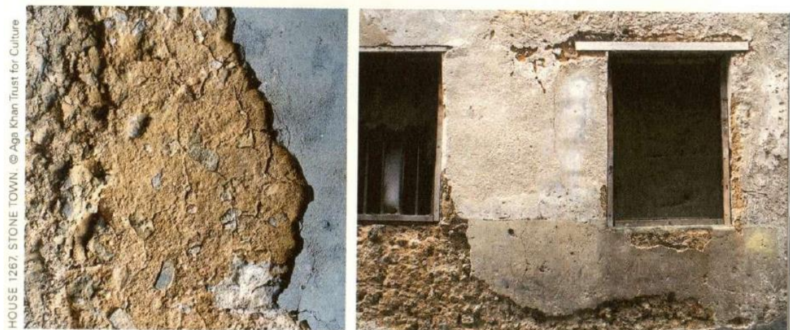
Figure 3-26 Identification of cement as an inappropriate restoration material, from Battle, Melin, and Forsman 2007
