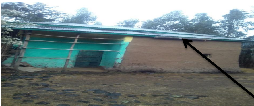
Fig 3.4 Traditional household rainwater collection system
