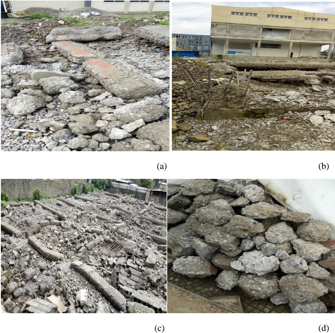
Fig. 3. 1Demolished site (a), (b) & (c) and collected demolished concrete (d)
