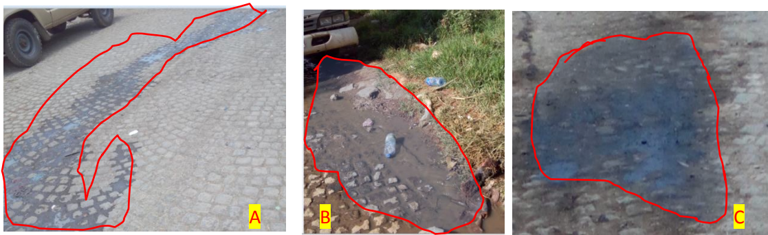
Figure: 4.64 :pollution of Cobblestone roads by liquid and solid wastes
