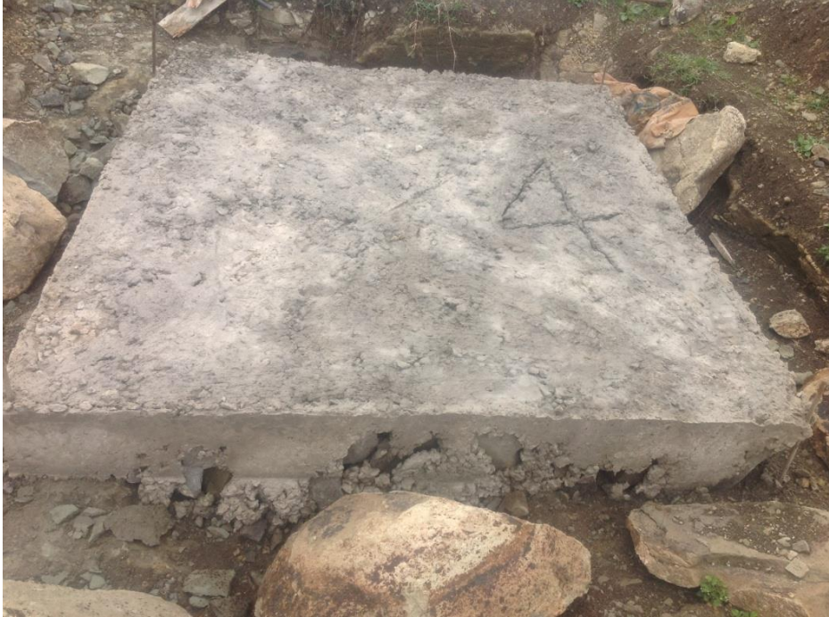
Figure 15 28 days Concrete Sample #4 ( 6cm concrete thickness with no wire mesh )
