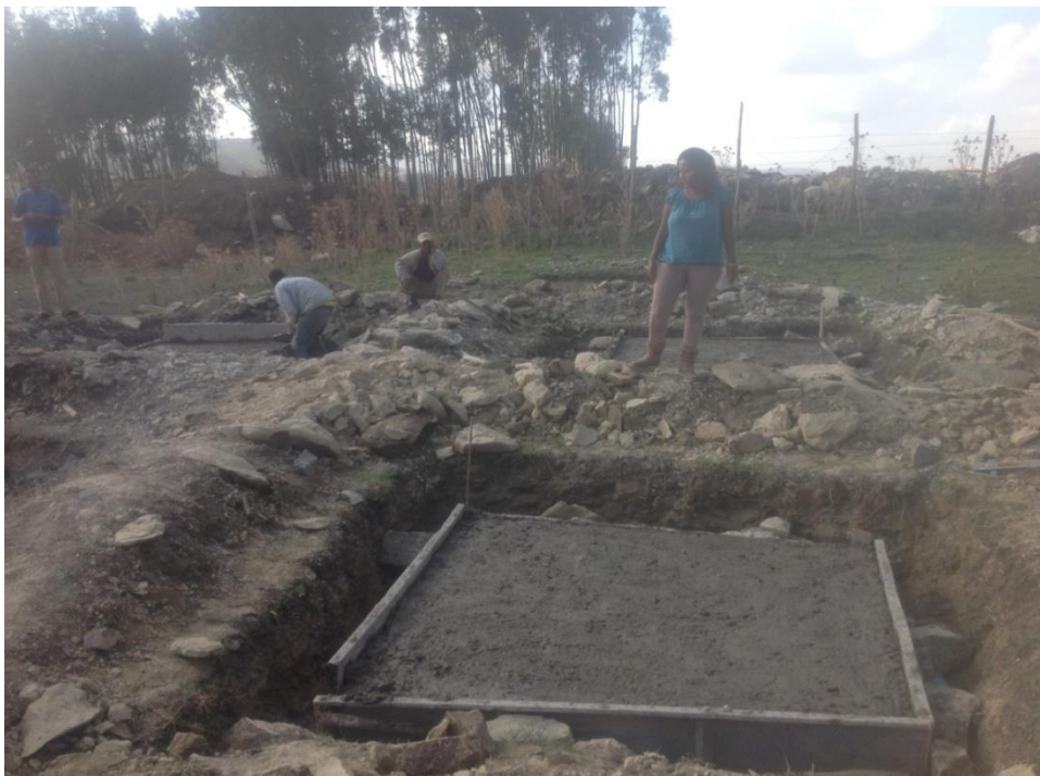
Figure 10 Fresh Concrete Cast of Sample #4 (6cm concrete thickness with no wire mesh)
