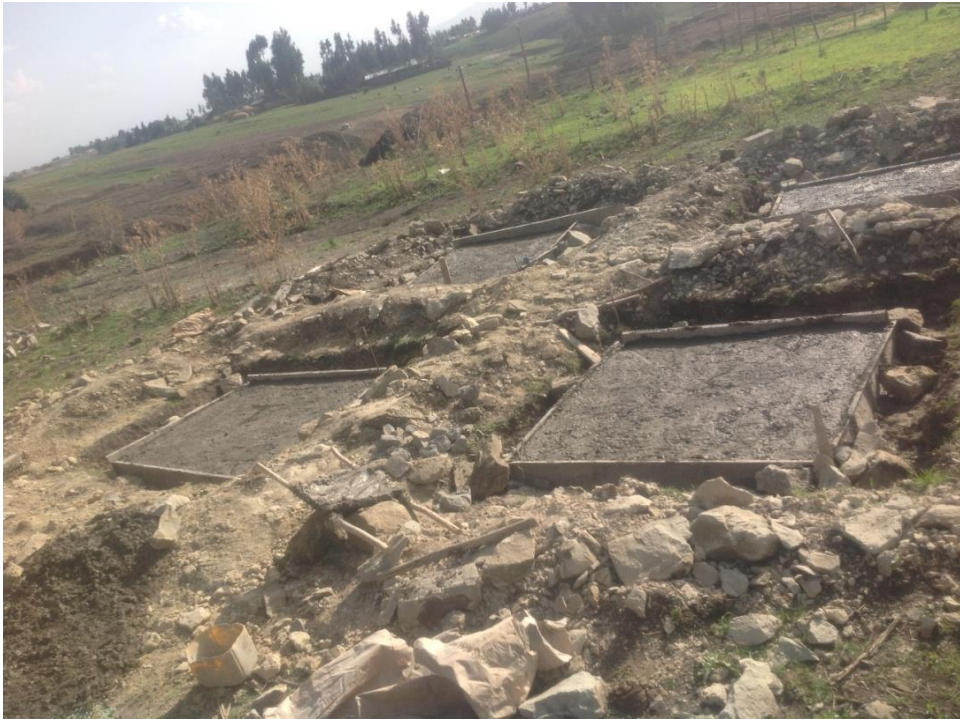
Figure 11 Fresh Concrete Caste of All Sample #1 - #4
