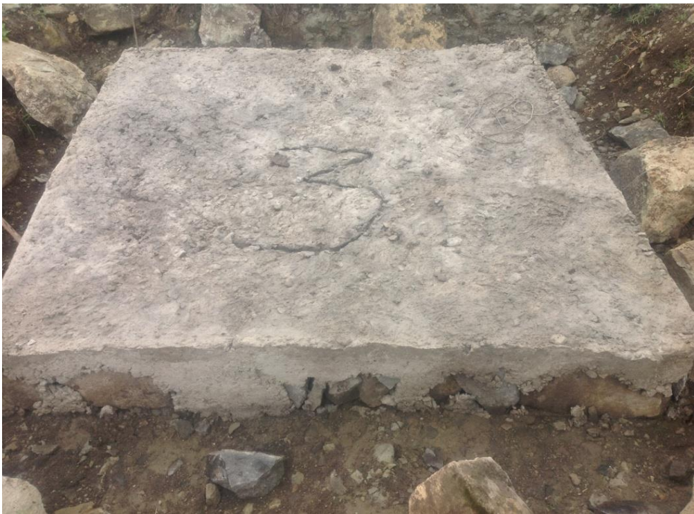
Figure 14 28 days Concrete Sample #3 (8cm concrete thickness with no wire mesh)
