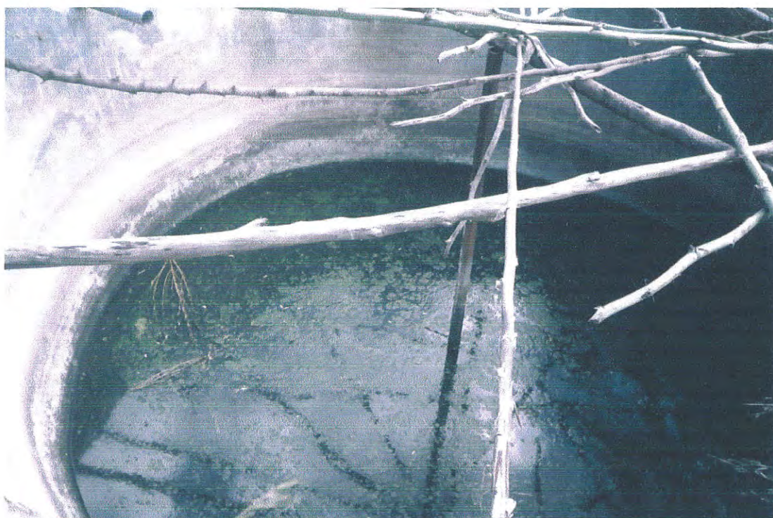
Picture 5.6: Accumulation of Plant remains in the Upper surface of the RWH Structure in Abecho kebele, March 2005.
