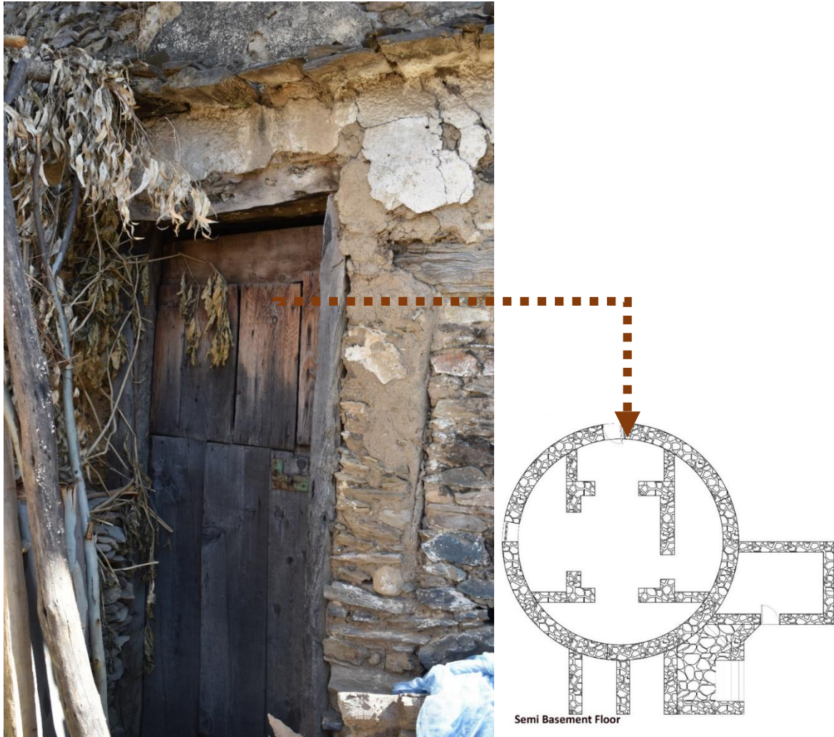
Figure 9: Wall altered to introduce a new door
