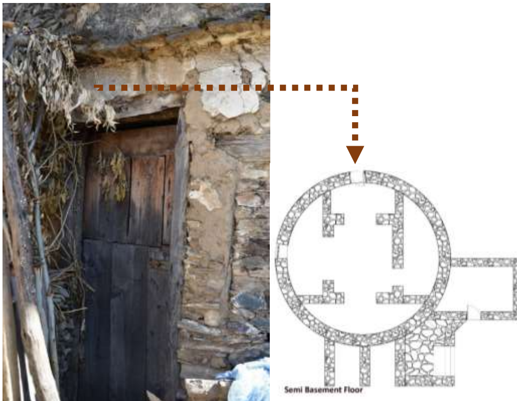
Figure 13: Wall altered to introduce a new door
