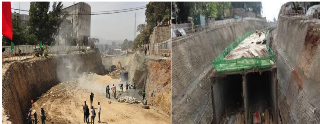
Figure 12 Menellik II tunnel construction.
