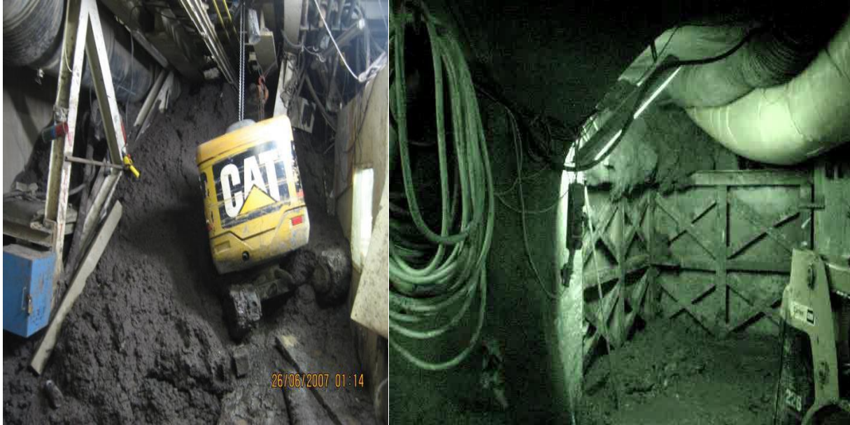
Figure 17 Extracting of mud: a) from the power tunnel b) from exploratory Adit. [4]
