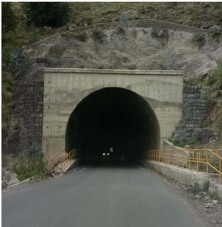
Figure 13 Tarmaber tunnel after maintained
