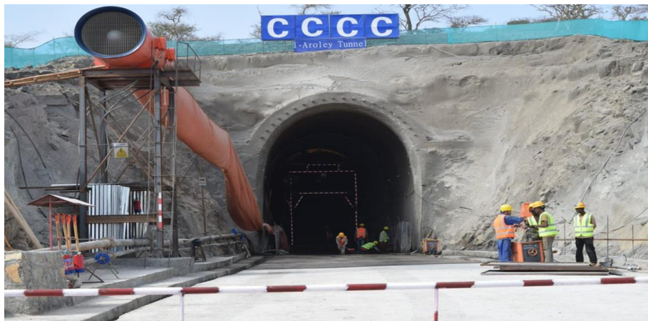
Figure 11 Aroley railway tunnel
