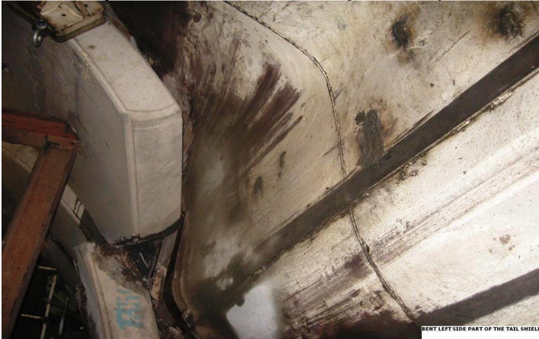
Figure 14 Tail TBM shield damaged and bent [4]
