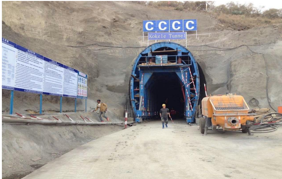
Figure 10 Kokele railway tunnel
