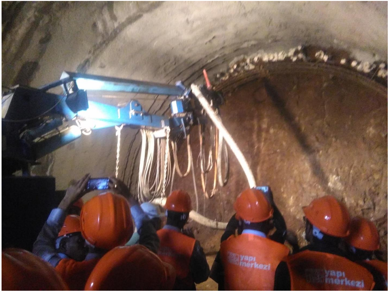
Figure 5 Visiting Tunnel construction at AKH railway project
