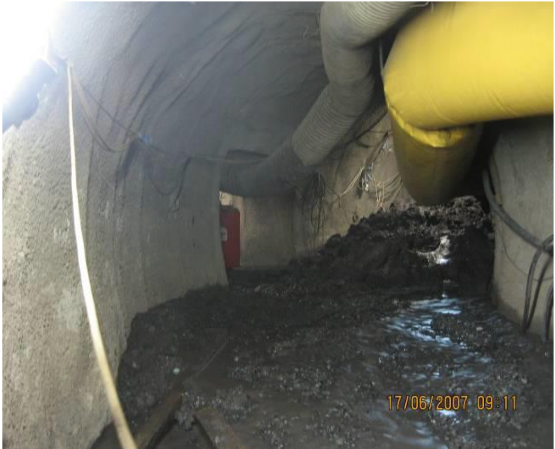
Figure 16 Mud in the Exploratory Adit [4].
