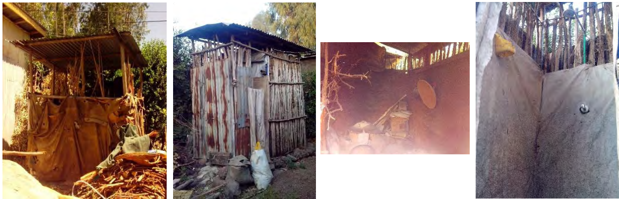
Figure 4. 9 Toilet, shower and traditional kitchen as detached units from the main house
