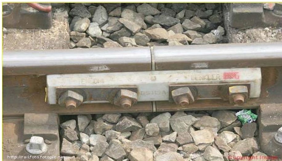
Figure 1.4: Symmetrically suspended rail joint [10]
