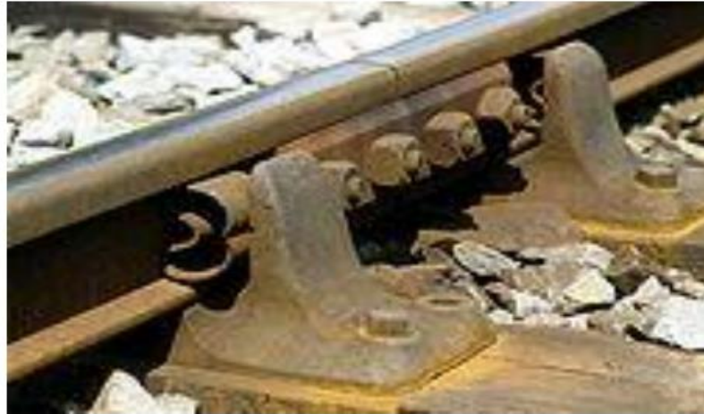
Figure: 1.3 a typical rail joint [15]
