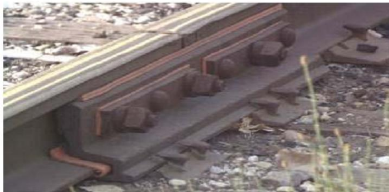
Figure1.9: Continuously supported joints on sleepers [13]
