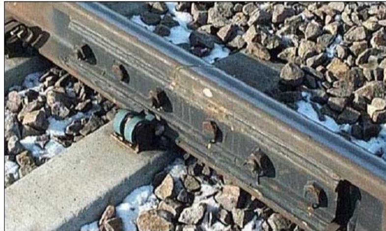
Figure 1.6: Discrete concrete sleeper supported joint [11]
