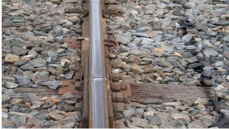
Figure1.7: Discretely supported joint on a timber sleeper
