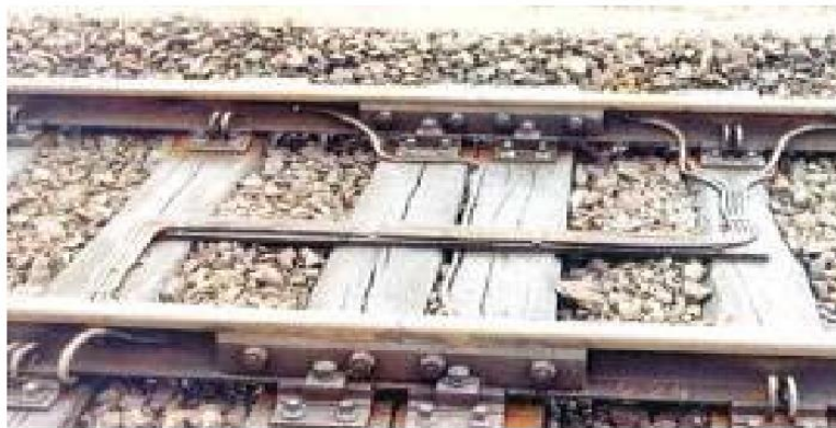
Figure1.8: Supported joint on two timber sleepers [12]
