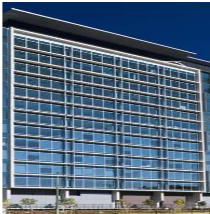
Figure 2-2: Window walls
