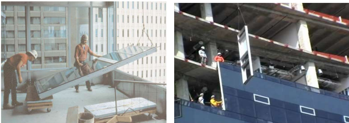
Figure 2-5: Unitized (unit panel) curtain wall system
