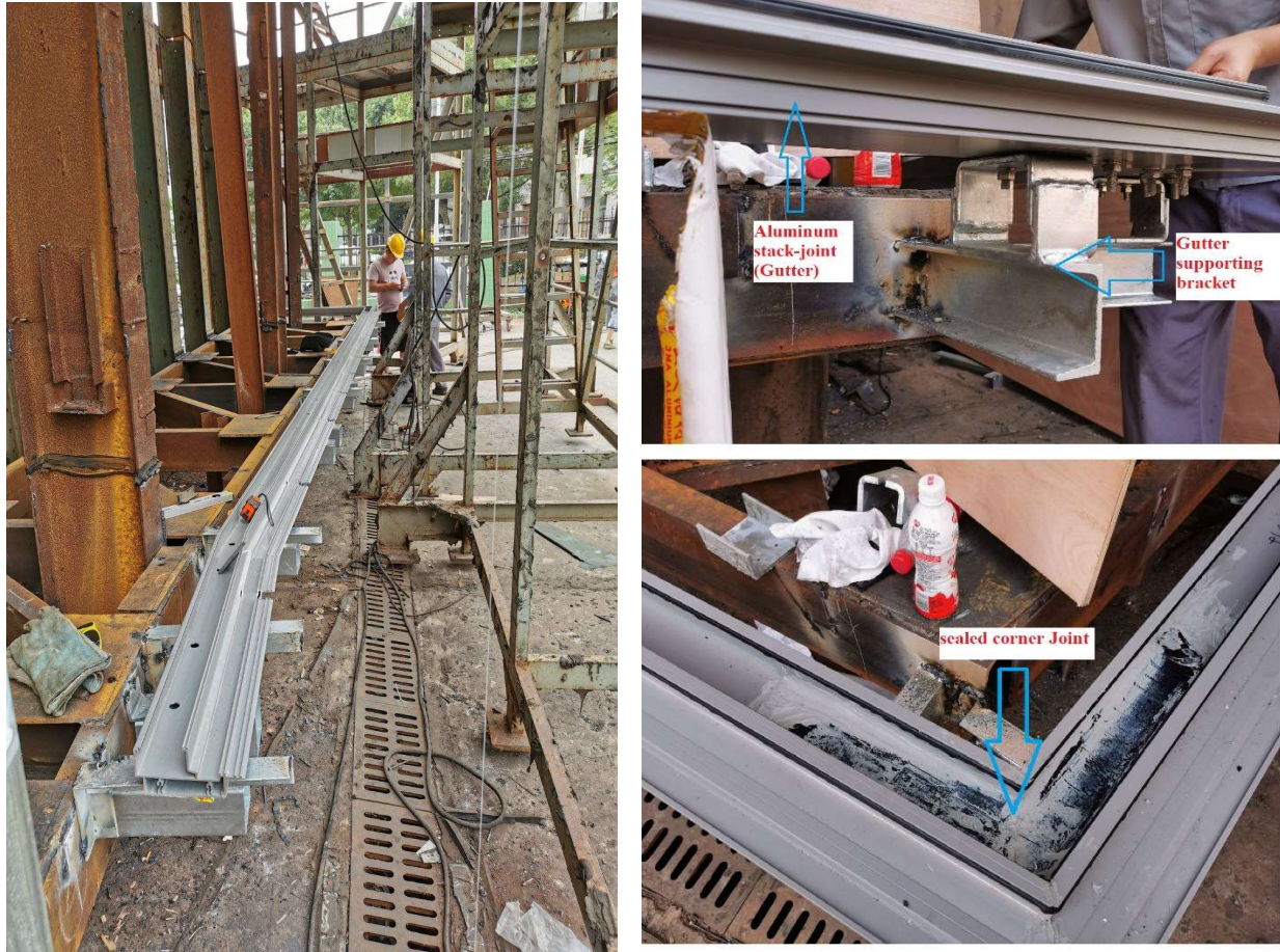
Figure 5-4: Bottom Gutter fixing and weather sealing
