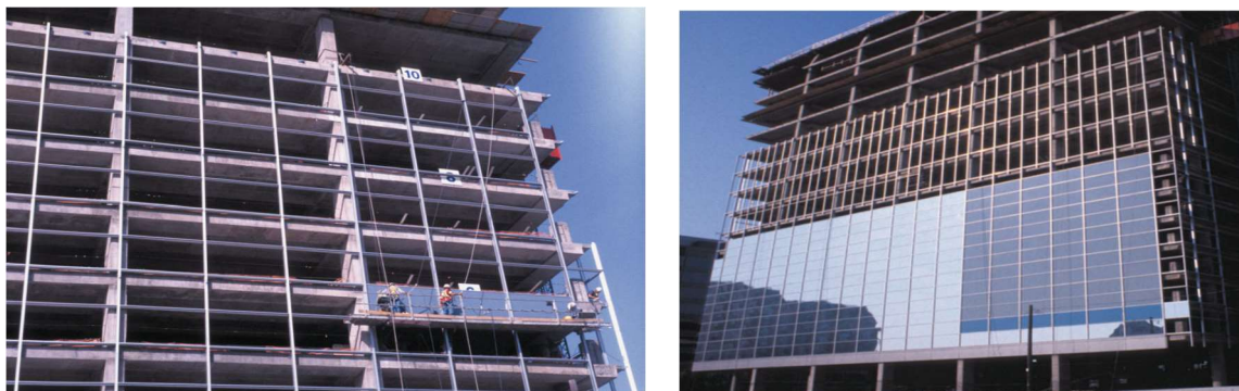
Figure 2-4: Stick-built curtain wall
