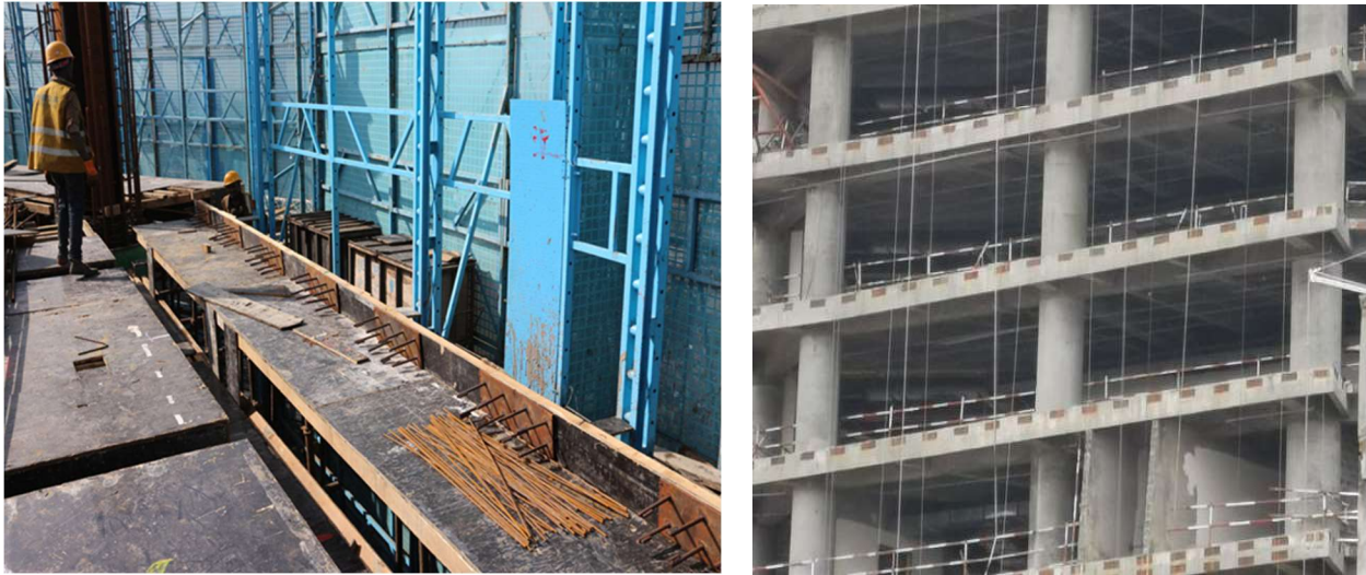
Figure 4-17: embedded plate anchorage for curtain wall support
