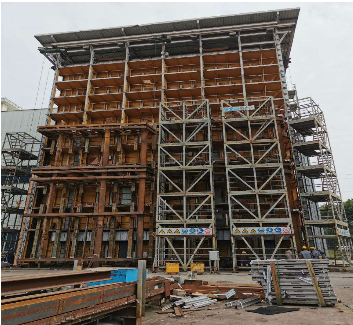
Figure 5-1: Curtain wall testing chamber
