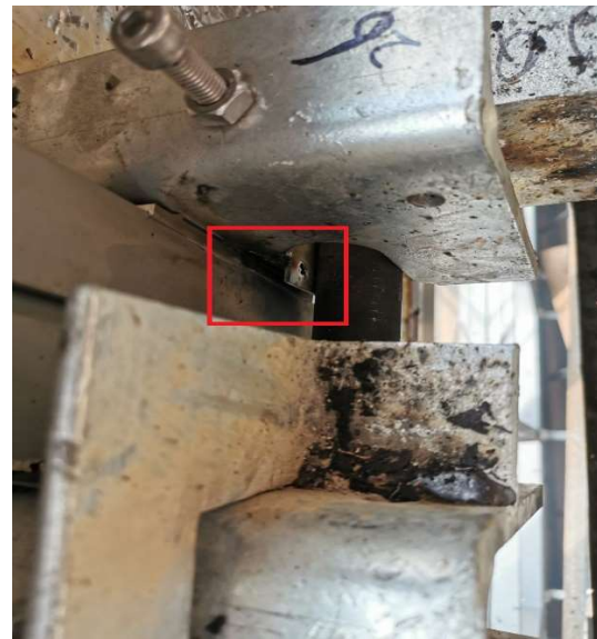
Figure 6-13 Additional steel plate inserted on the gap as a modification
