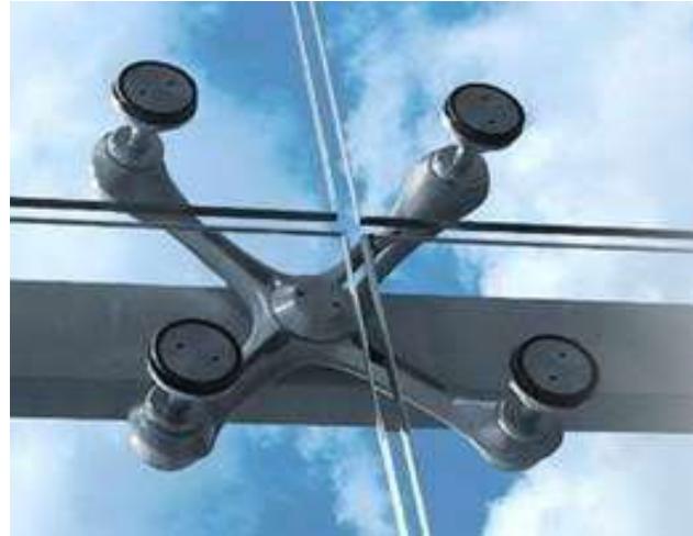
Figure 2-12: Point-fixed structural glass façade system
