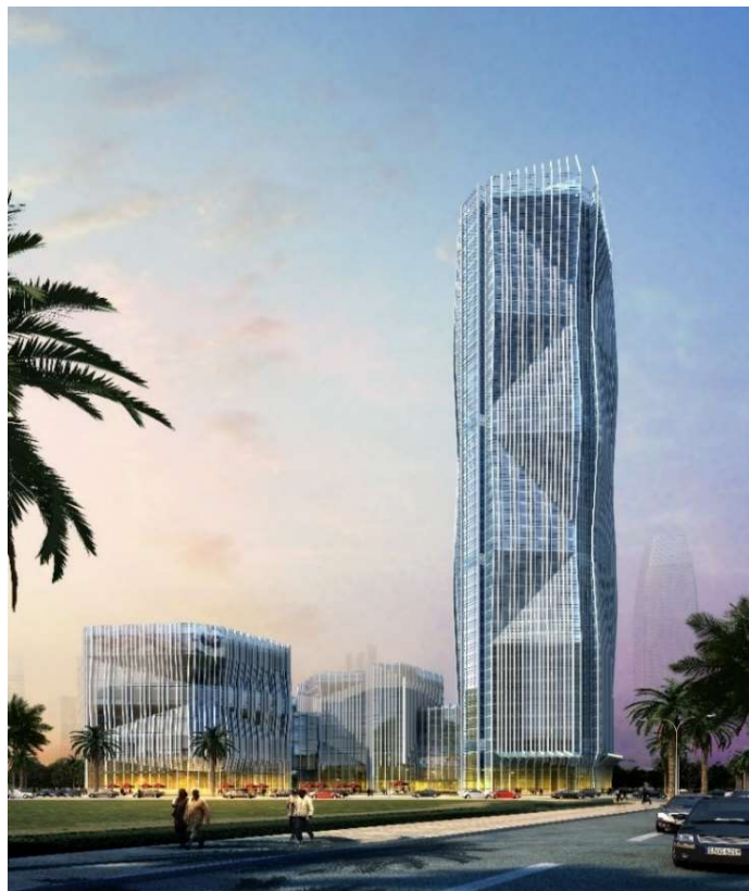
Figure 4-1: CBE HQ Building
