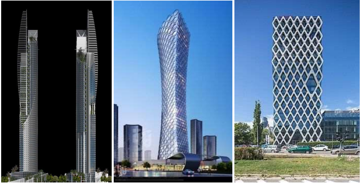
Figure 3-2: High-rise buildings curtain wall facades
