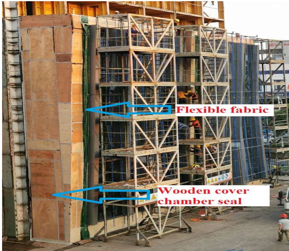
Figure 5-8: Chamber sealed using wooden cover and flexible fabric
