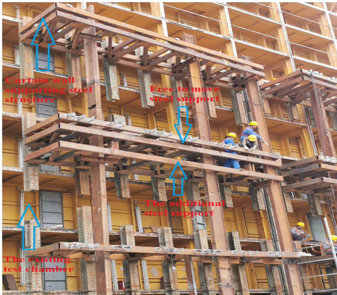
Figure 5-21: Curtain wall test specimen supporting steel structure
