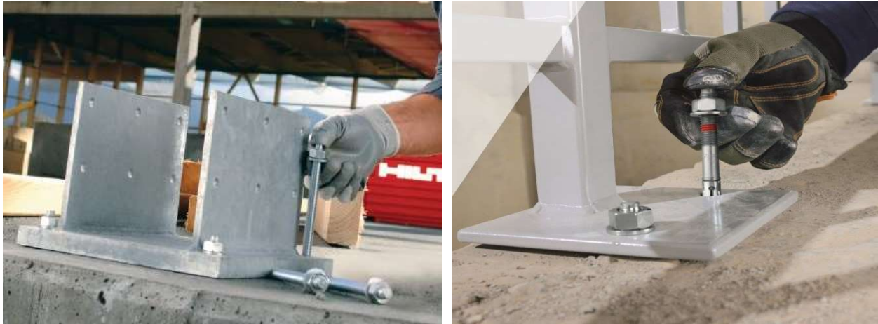
Figure 2-27: Anchor bolt anchoring system
