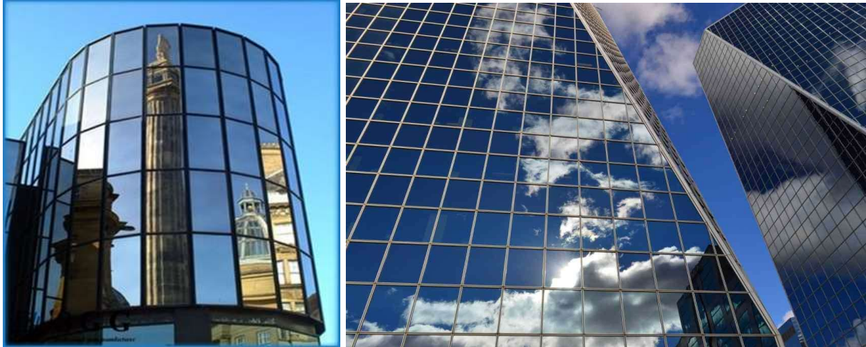
Figure 2-46: Reflective glass curtain walls
