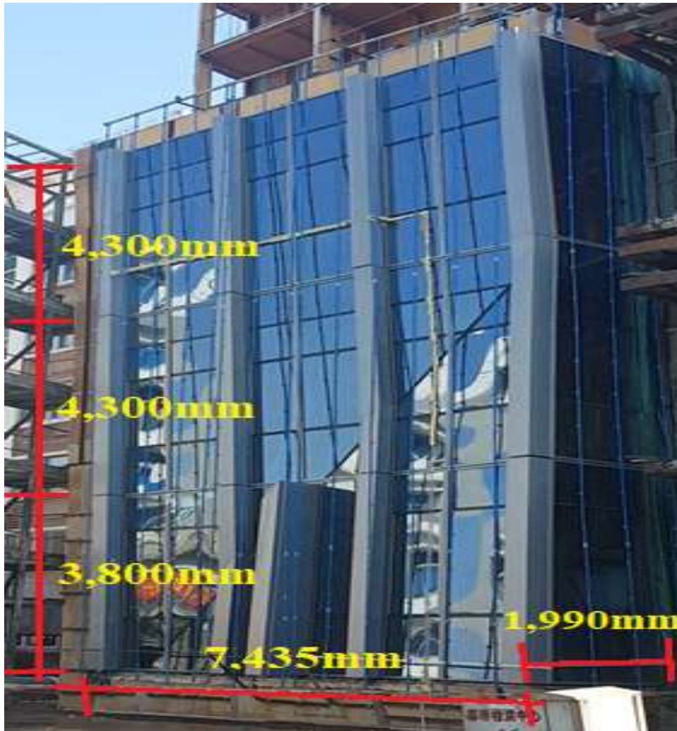
Figure 5-2: Curtain wall installed test specimen
