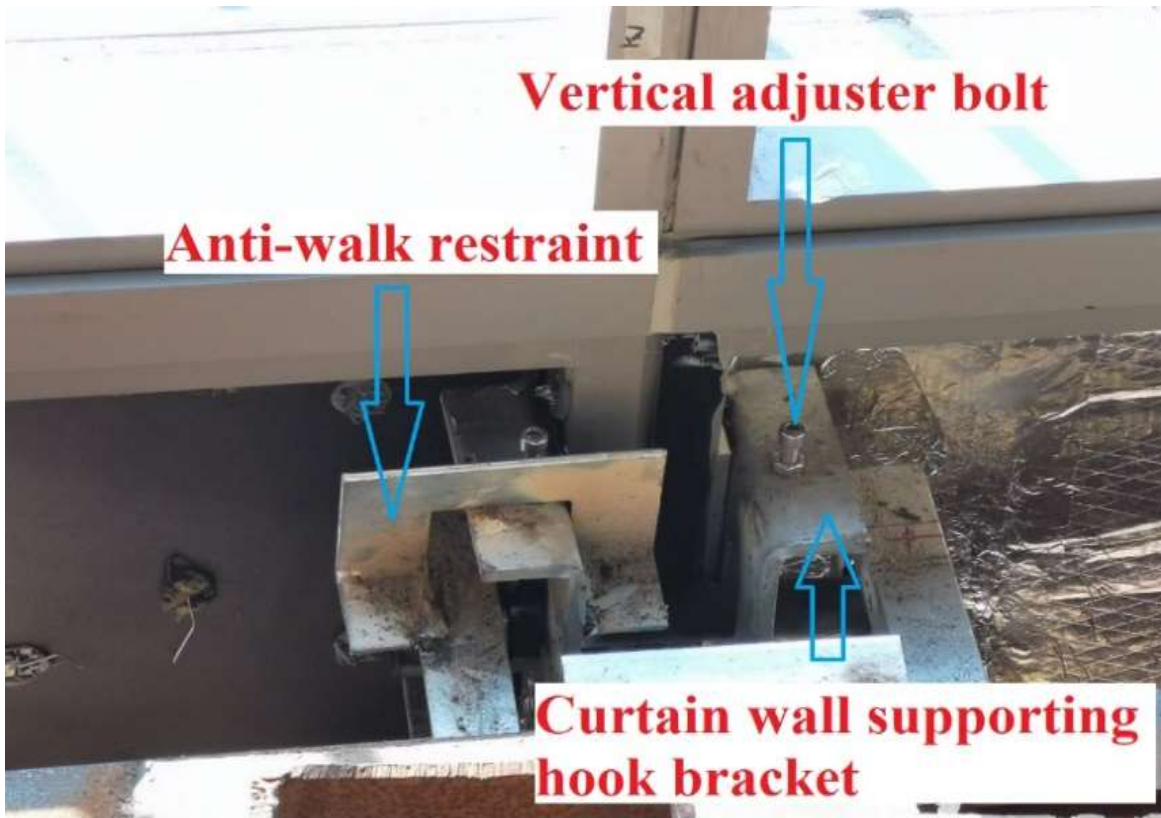
Figure 5-7: Anti-walk used on curtain wall supporting hook
