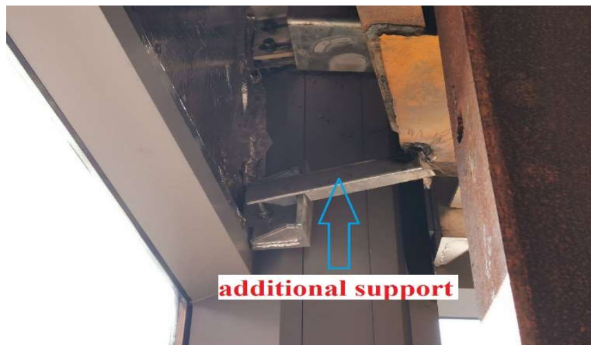
Figure 5-6: Additional supporting bracket
