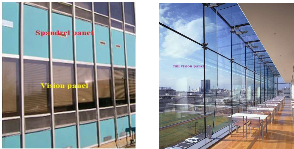
Figure 2-15: Vision and spandrel panel
