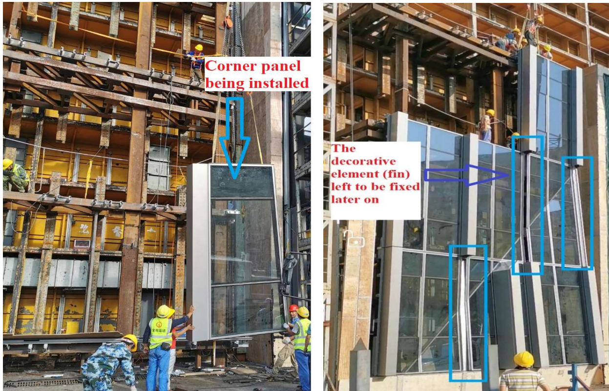
Figure 5-5: Unitized curtain wall test specimen installation
