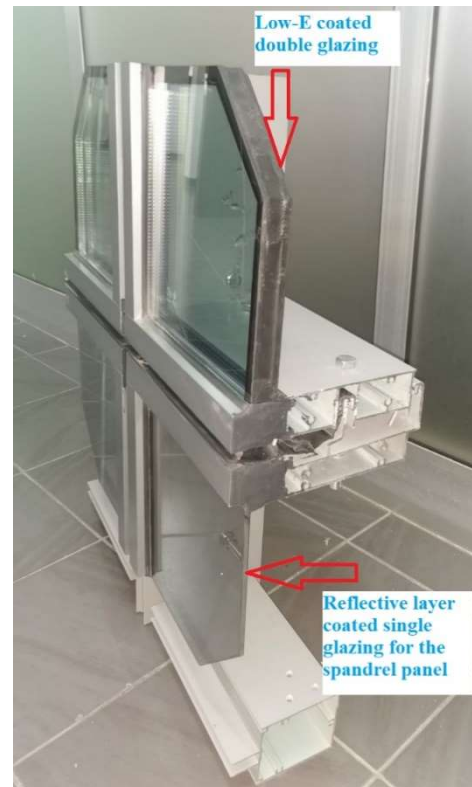
Figure 4-10: mini-sample of vision and spandrel panel glasses
