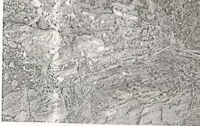
Figure 7.2. Jointed and fractured rock on the reservoir flanks
