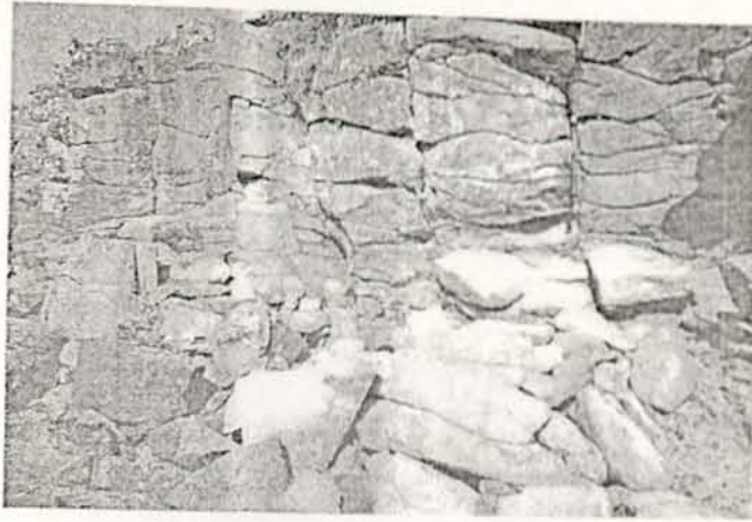
Figure 5.2. Orthogonal joint sets at the riverbank
