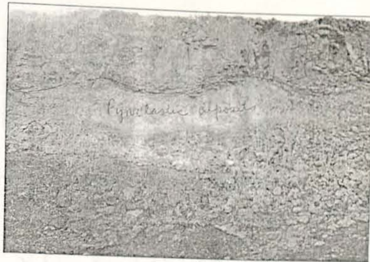
Figure 3.7. Friable pyroclastic deposits at the dam site
