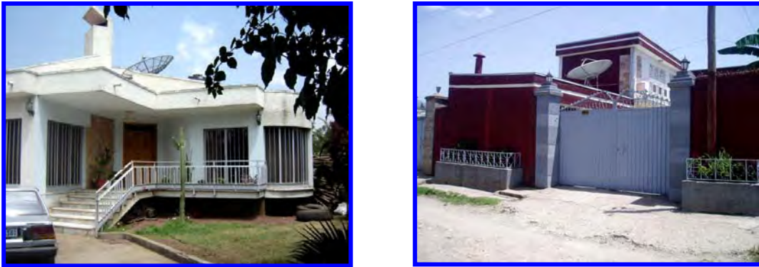
Fig 6.3. New Informal settlements built from standardized materials in Reppi Areas
