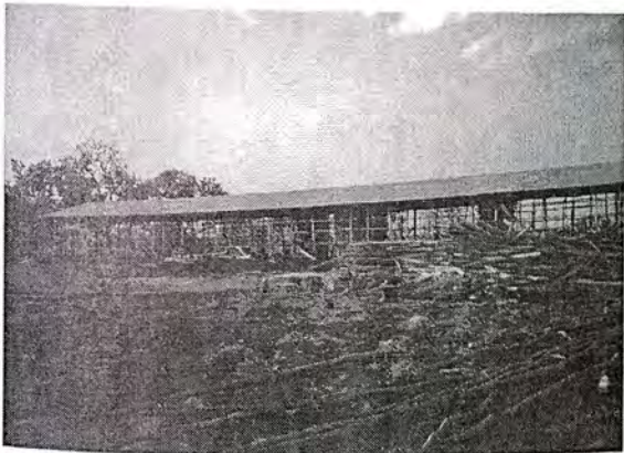
15. A new school under construction by the regional government
