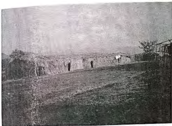
19. School built by the settlers' community
