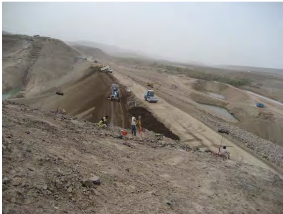
Figure3.1: Cofferdam under construction
