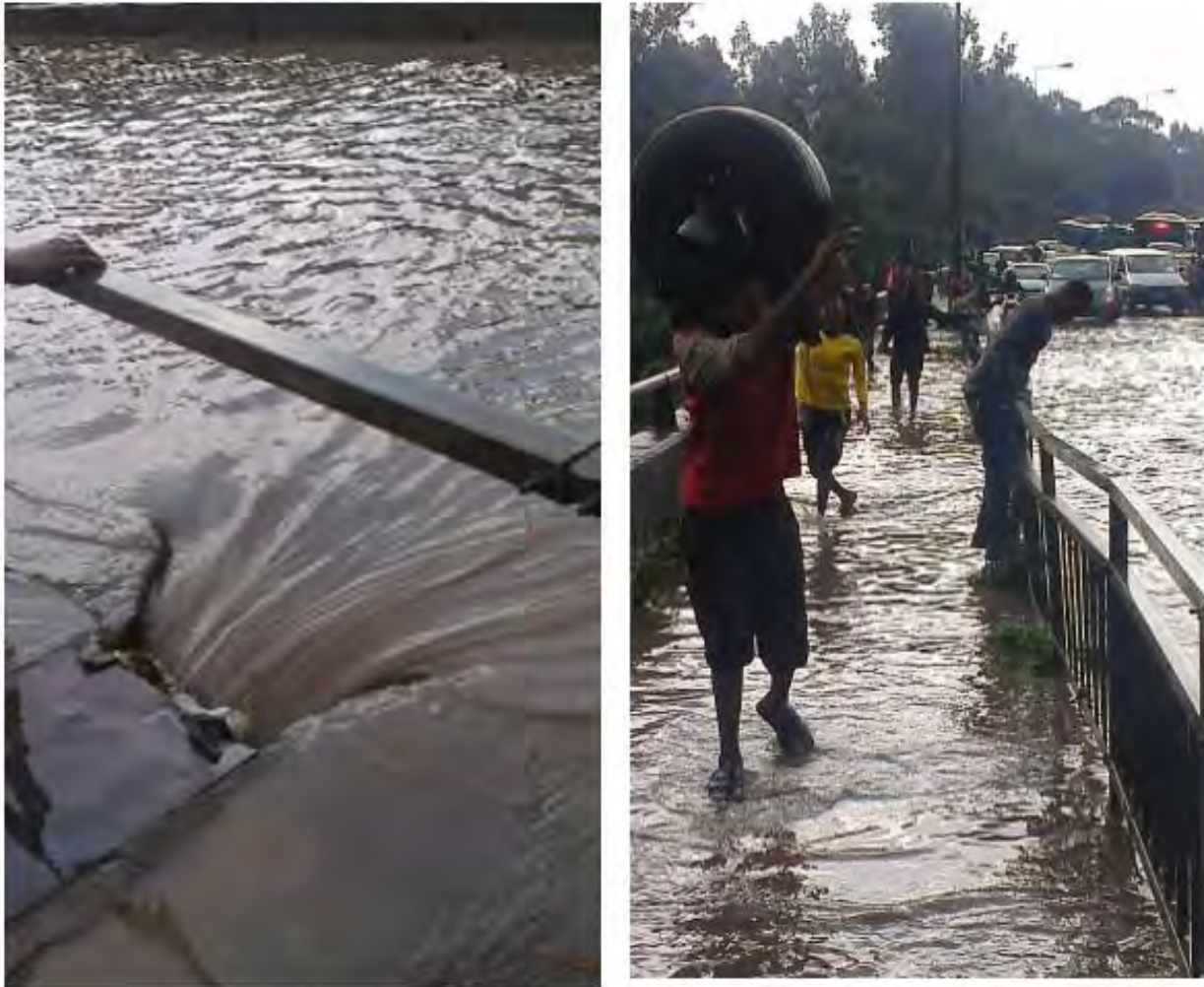
Figure 1: Left- Storm Water escaping into a river through an illegally widened inlet at the side of bridge. Right: Both main asphalt road and walk way flooded
