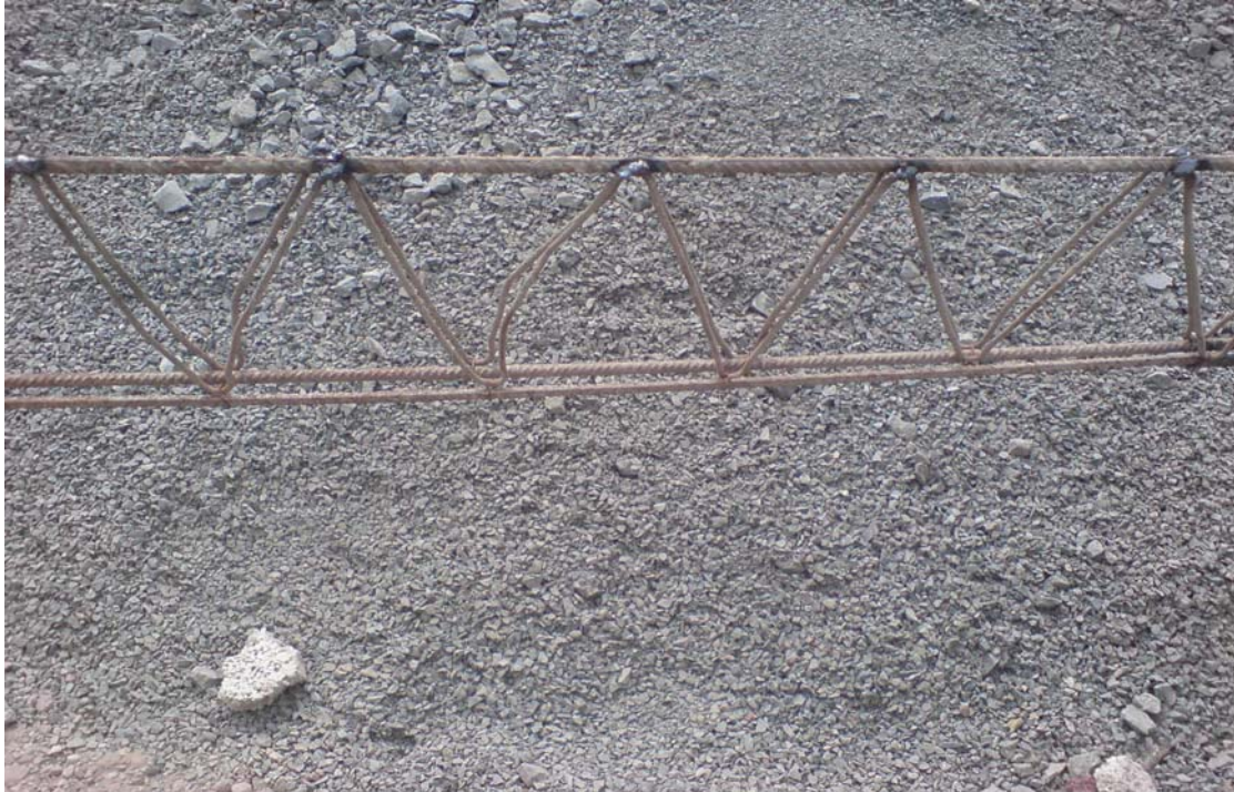
Fig1.9 Reinforcement welded at all nodes.
