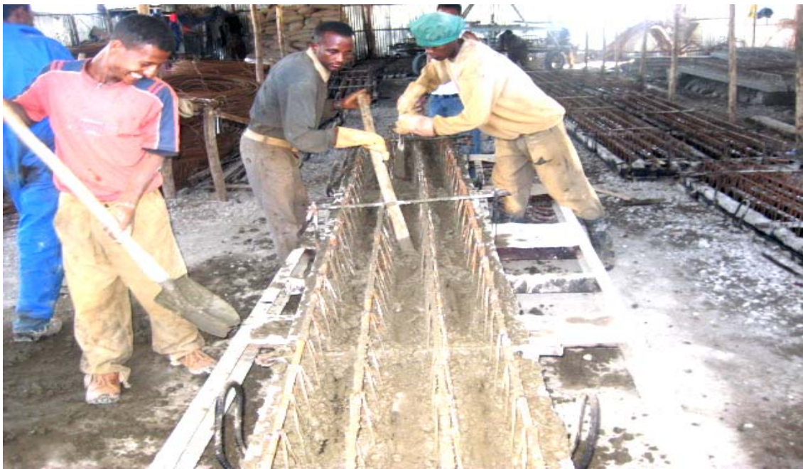
Fig. 2.7 Concrete Placing.
