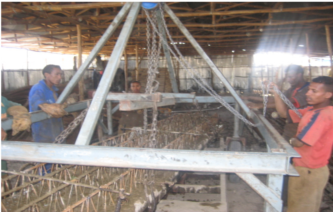
Fig. 2.9 Transporting using manual cranes.
