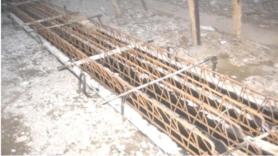
Fig. 2.6 Reinforcements welded and put in the mould.
