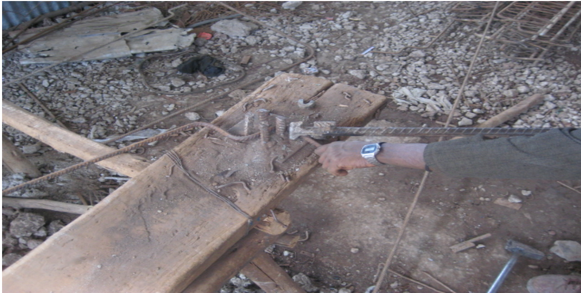
Fig.2.4 Bending of the main reinforcement.
