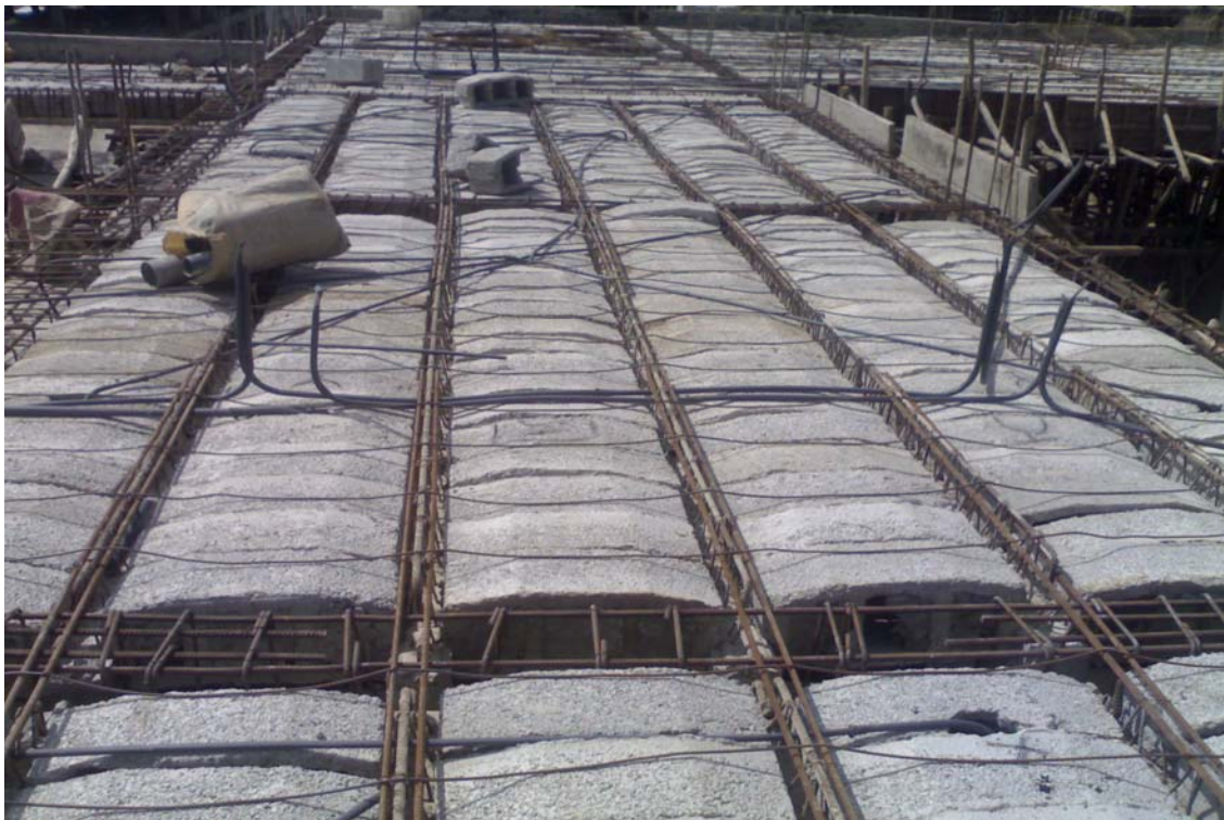
Fig1.10 Pre-cast Beam-Slab prior to concreting.
