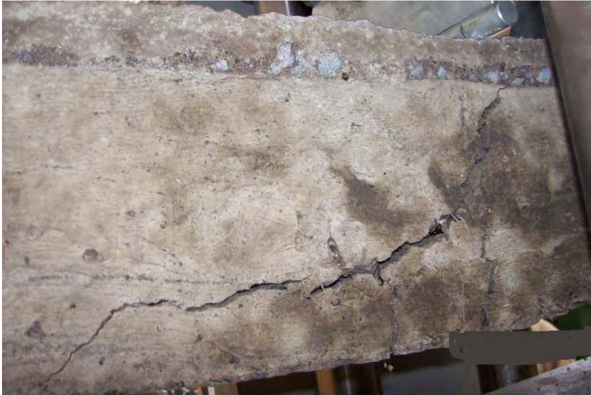
Figure 4.5 Failure pattern for F-treated, 2.5-1
