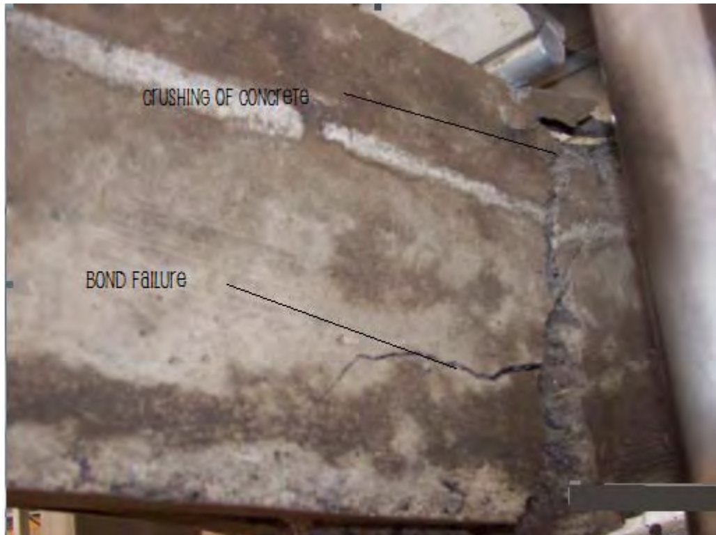
Figure 4.4 Failure pattern for F-treated, 2.5-1
