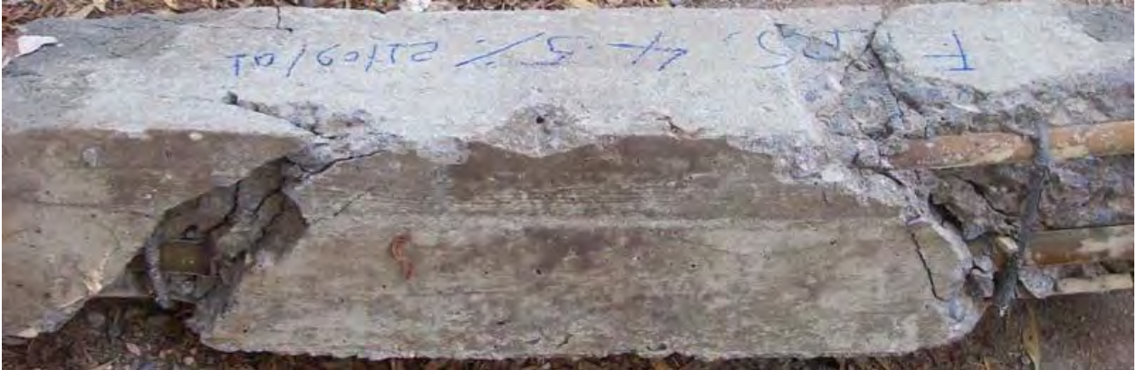
Figure 4.13 Failure pattern for F-untreated, 4.5-10
