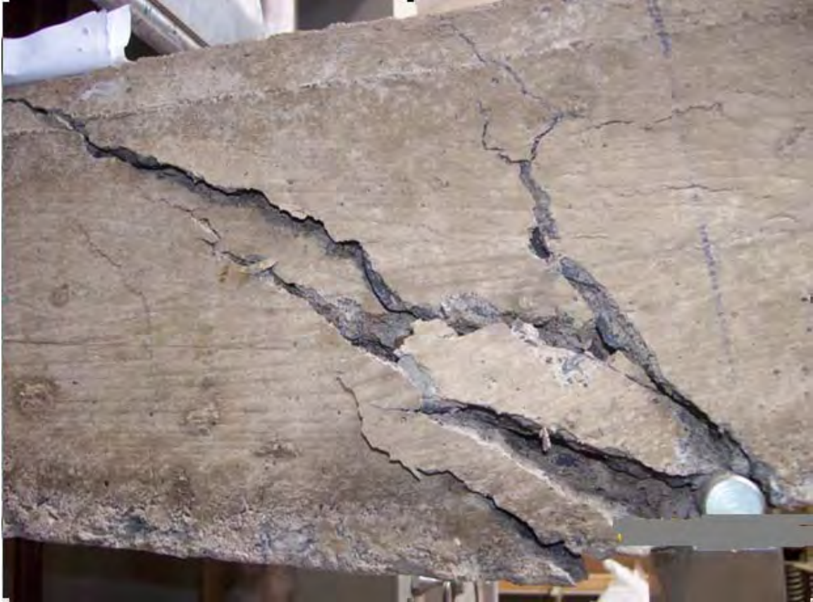
Figure 4.11 Failure pattern for F-untreated, 3.5-8
