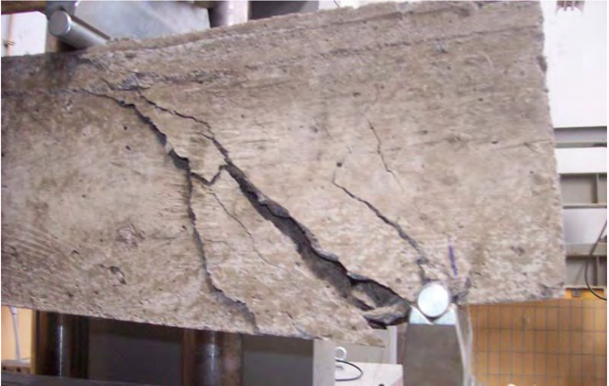
Figure 4.10 Failure pattern for F-untreated, 3.5-7
