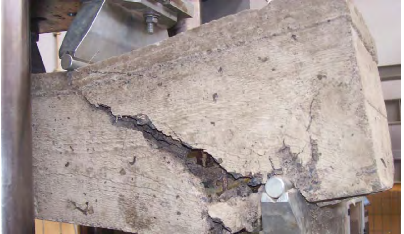
Figure 4.14 Failure pattern for F-untreated, 4.5-11
