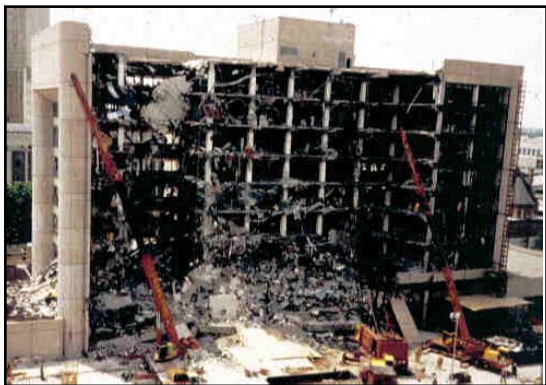
(a) Alfred P. Murrah Federal Building
