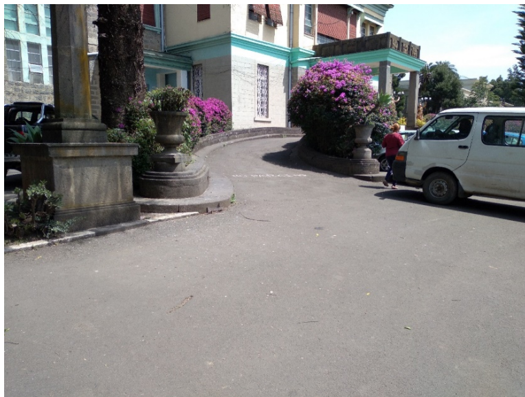
Fig. 32. One of the Ramps built at the building entry of the Institute of Ethiopian studies (Photo taken in 2021 by Abrham Tesfaye).
