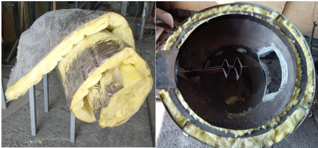
Figure 37: Applying Fiber Glass Insulation
