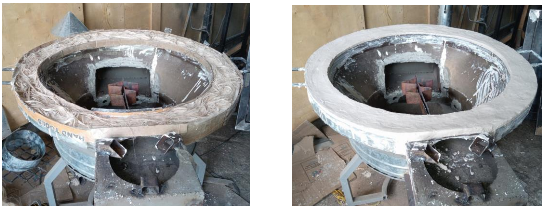
Figure 38: Preparation and Applying Gypsum
