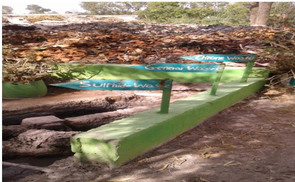
Figure:-7. Wastewater segregation lines and a partial view of heap of solid waste, Modjo tannery
