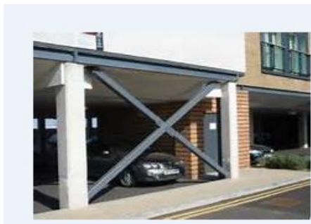
Figure 2.3: Internal bracing
