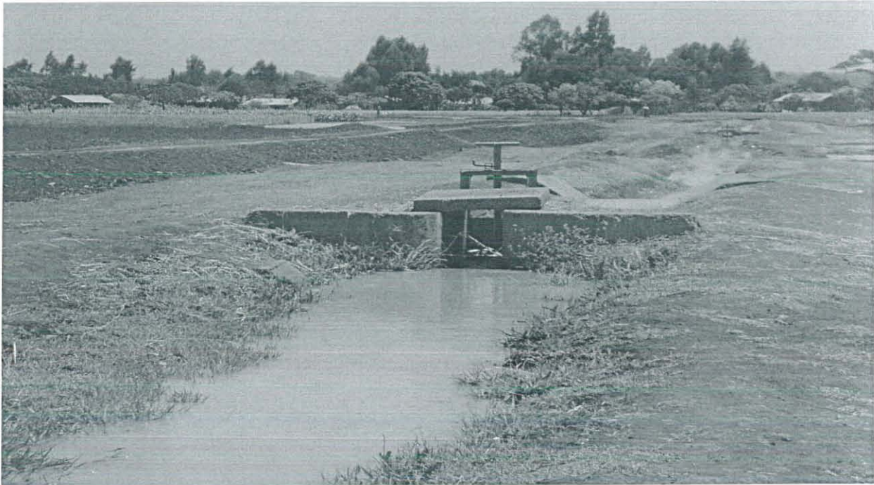
Figure 5: Unlined Tertiary canal
