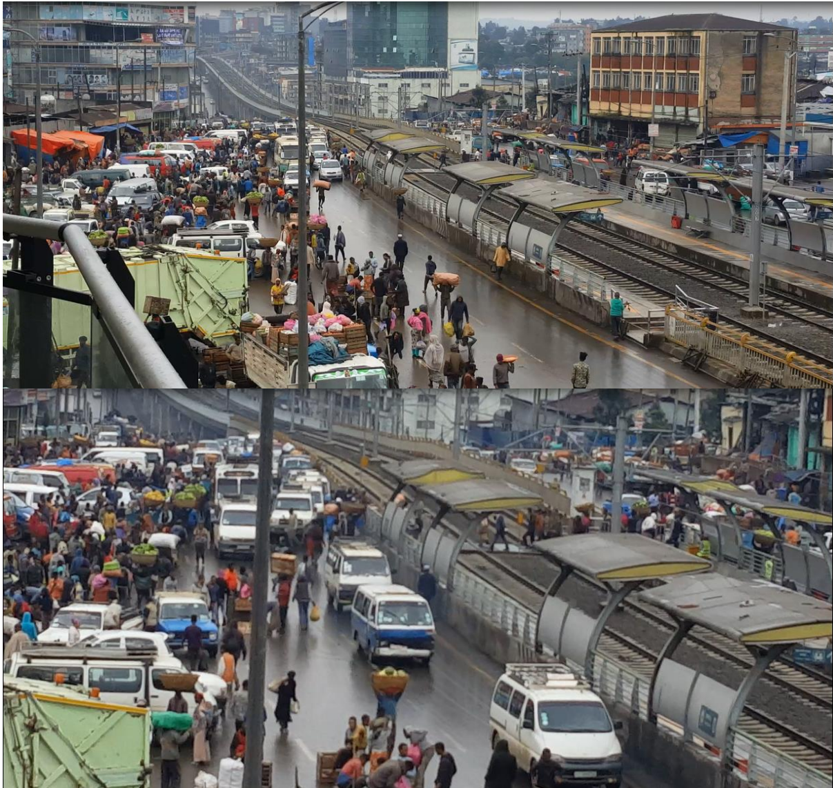
Fig 5. 19 Traffic congestion caused by absence of pedestrian bridge at ATKELT TERA.
