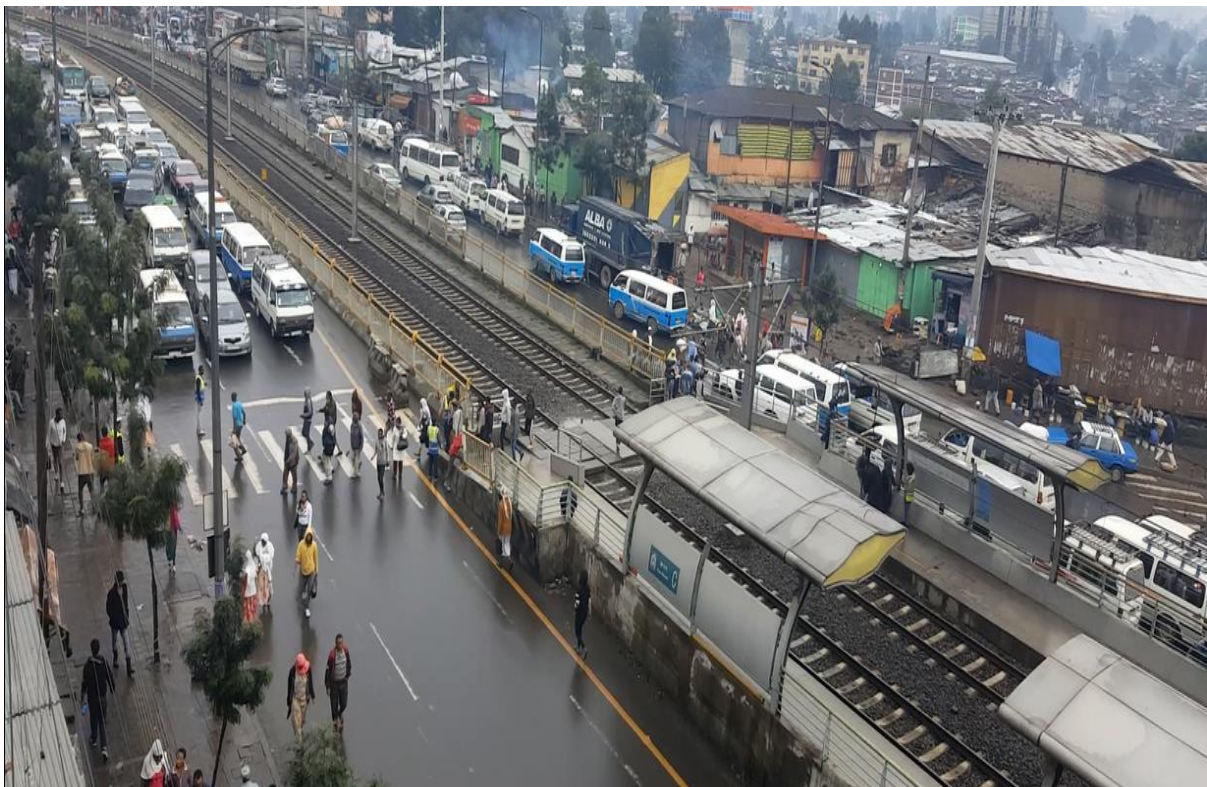
Fig 5. 18 Traffic congestion caused by absence of pedestrian bridge at ATKELT TERA.
