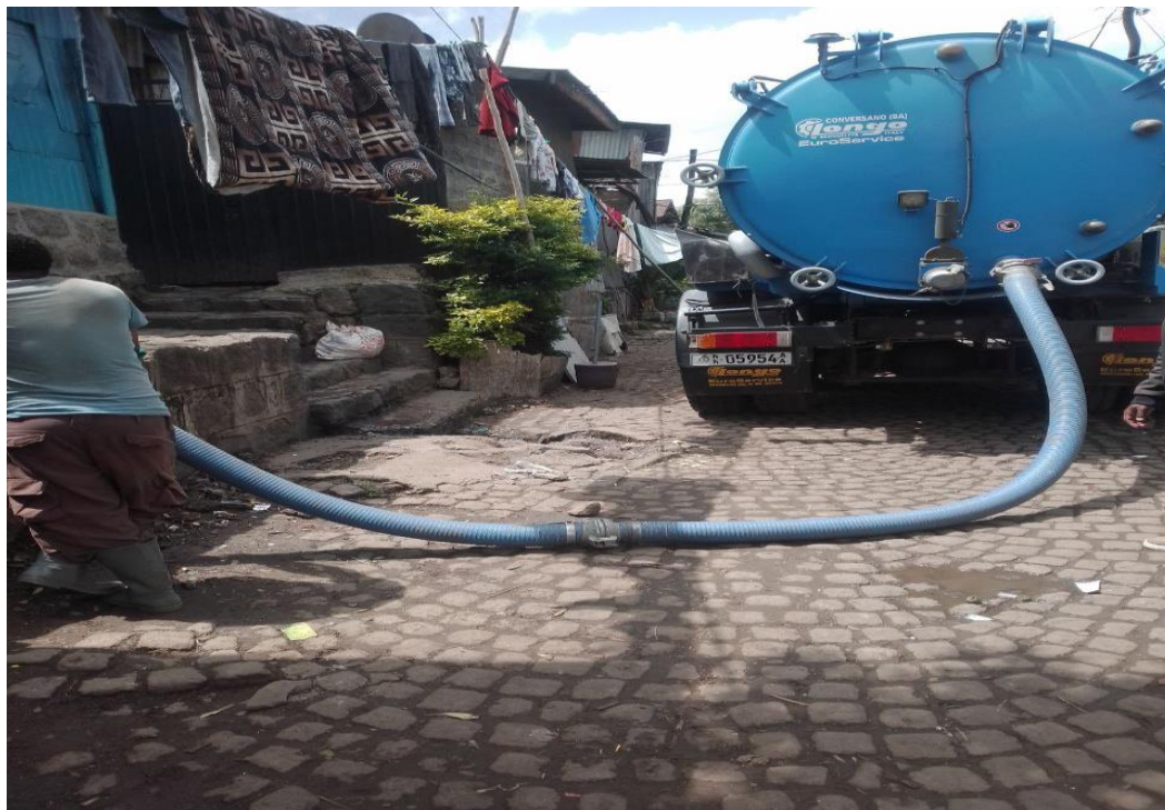
Figure 2. AAWSA Pit latrine Sludge when removed by vacuum truck around the Teklehaimanot area
